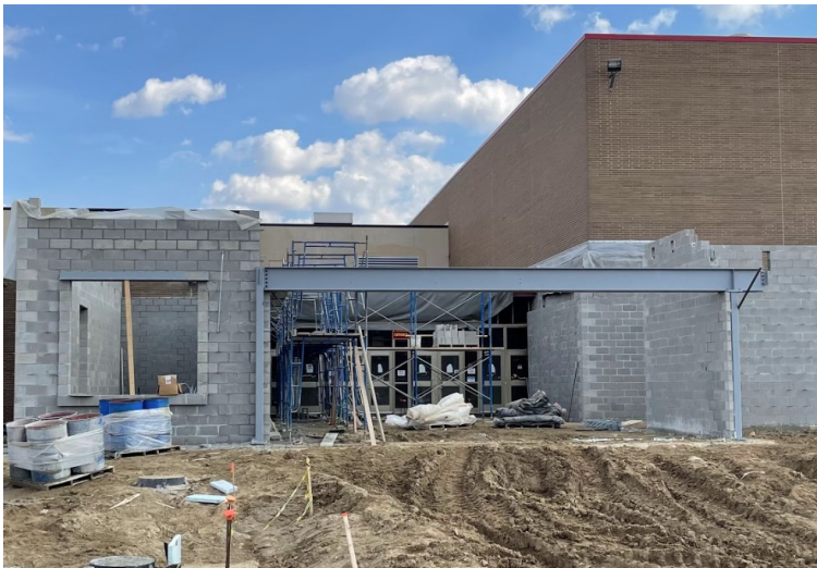
Block work continues on what will be the new main entrance on the west side of Davison High School.
