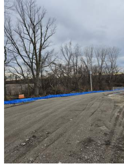
Temp Road (Asphalt Millings)
