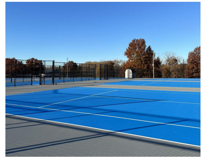
North Courts Looking Southwest
