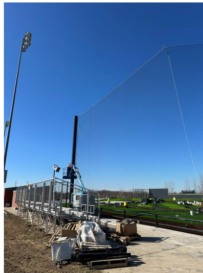
LNHS - Baseball (Backstop Netting Installed)
