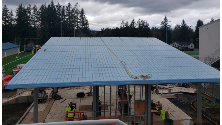
Lakeridge High School Outdoor classroom view from the cafeteria
