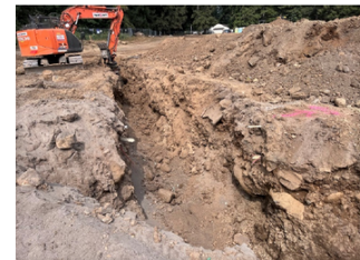
Backfill of existing utility trench
