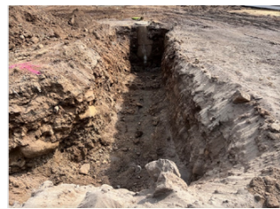
Removal of utilities
