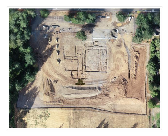
Contractor has been removing dirt and sand from previous building's site and stockpiling the material in preparation for the installation of compacted base material for the new building
