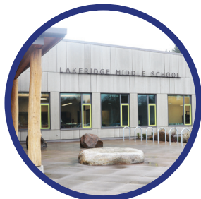
New building for Lakeridge Middle School
