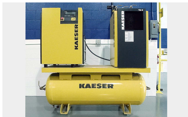
The shop compressor can supply Grade-D air, but there must be monitoring devices to detect contaminants installed.
