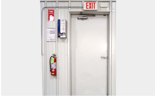
Exits must be properly marked.
