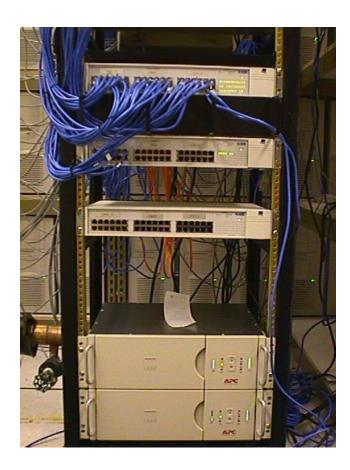
Intermediate Distribution Frame (IDF): A secondary hub in the network, typically located between the MDF and end-user devices. IDFs are used to reduce the length of cable runs to individual devices and often house networking equipment like switches and routers.
