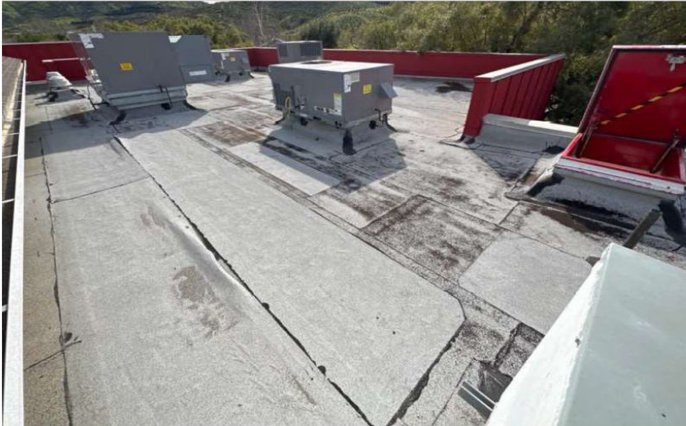
Flat roof- overview
