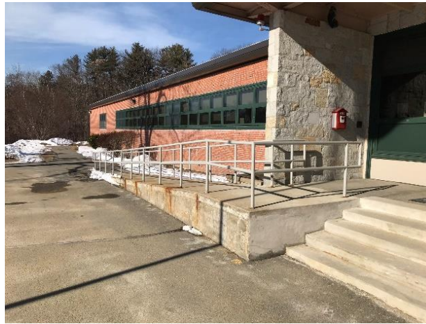
1.5 Non-Compliant handrails
