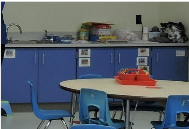
3.14 Classroom sinks are not wheelchair accessible
