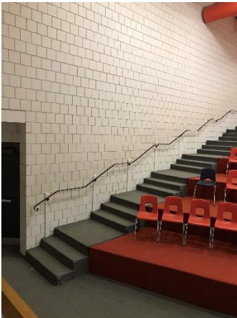
3.30 Handrail in the auditorium.
