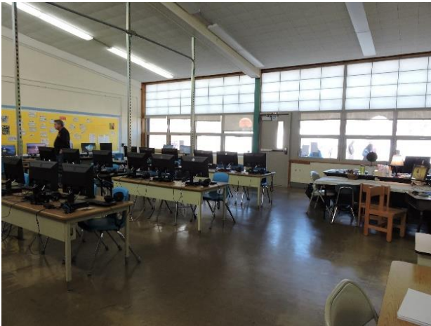
3.1 9"x9" asbestos floor tiles
