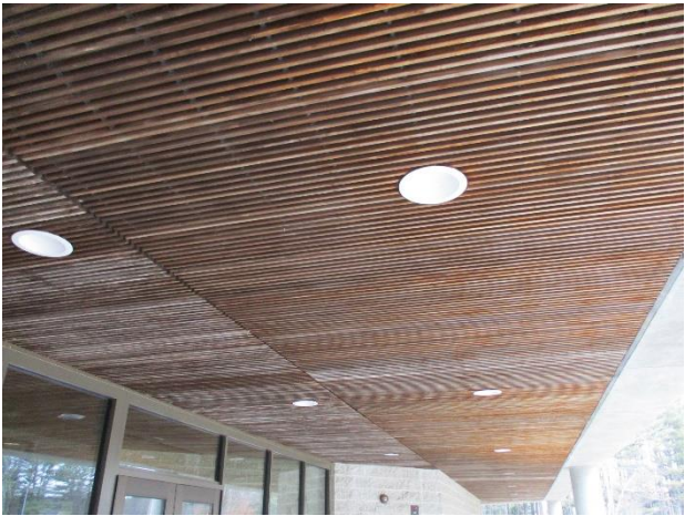
1.4 Overhang ceiling at main entrance.
