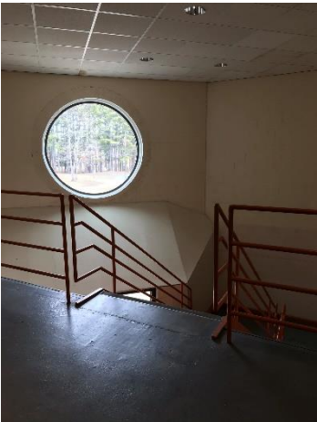
3.34 Handrails at Stair B.
