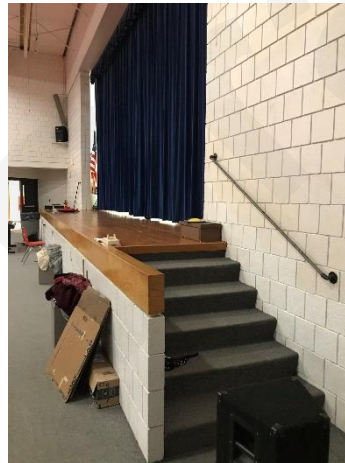
3.31 Handrail to the stage.
