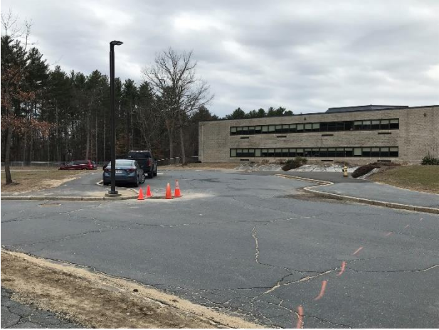
1.2 Bituminous paving at bus drop off.
