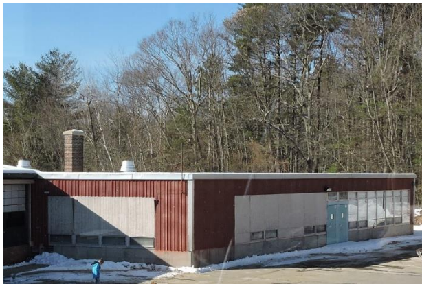
2.4 The abandoned 1960 addition
