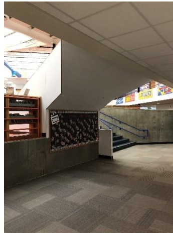
3.22 Underside of stair from library to second floor.
