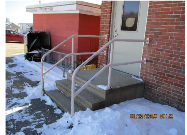
3.22 Gym egress stair
