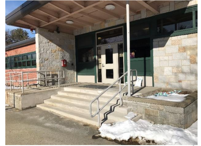
1.6 Canopy at main entrance
