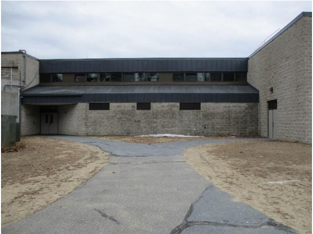
2.3 Sloped roof by the loading dock area.
