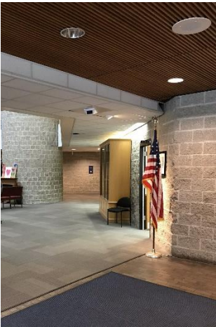
5.2 Security Camera and Intrusion Alarm System.
