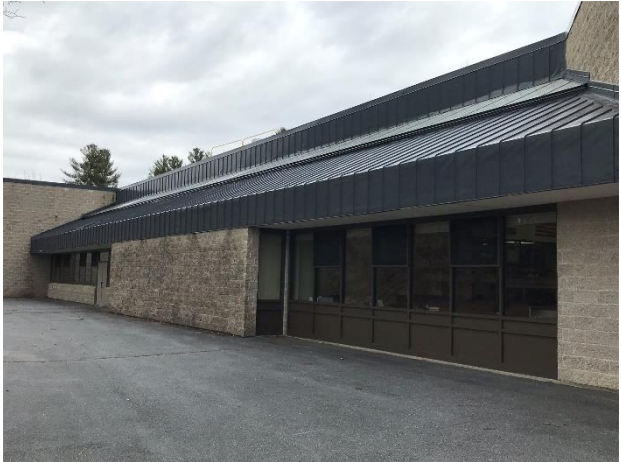
2.2 Sloped roof by the Music Room.
