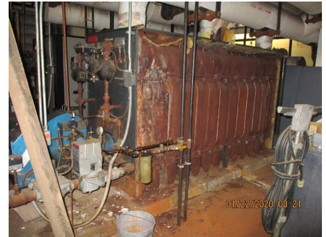
4.7 Non-functioning boiler
