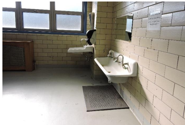
3.9 Toilet rooms in the 1950 building
