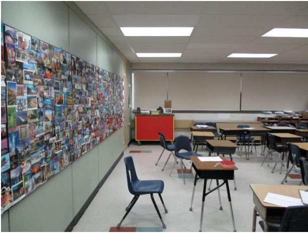
3.1 Demountable partition between classrooms.
