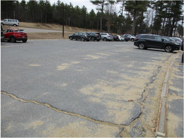
1.1 Bituminous paving at parking lot.
