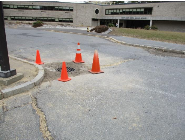
1.5 Newly replaced catch basin.
