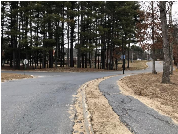
1.6 Granite curbs at bus drop off area.
