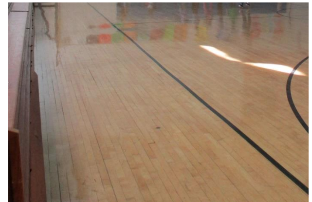
3.10 Gymnasium wood floor
