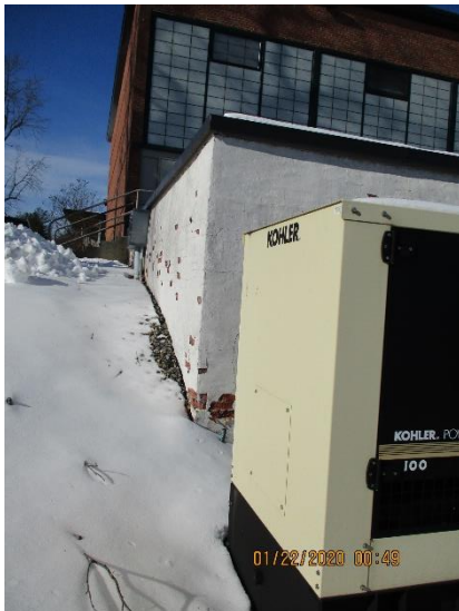
1.7 Exterior wall at electrical room
