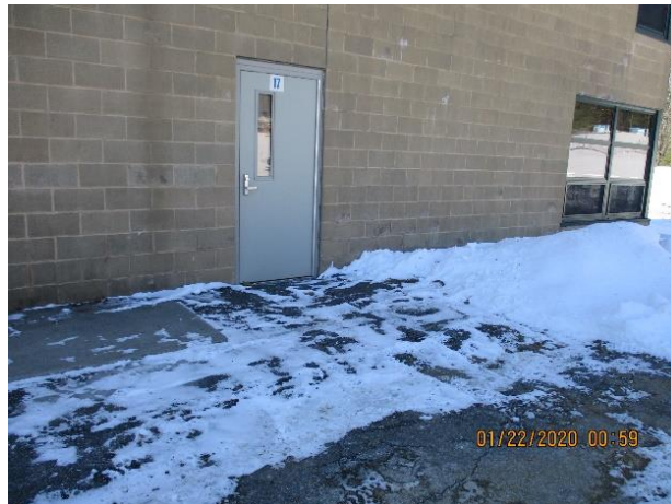
1.8 Bituminous concrete pad at exit door
