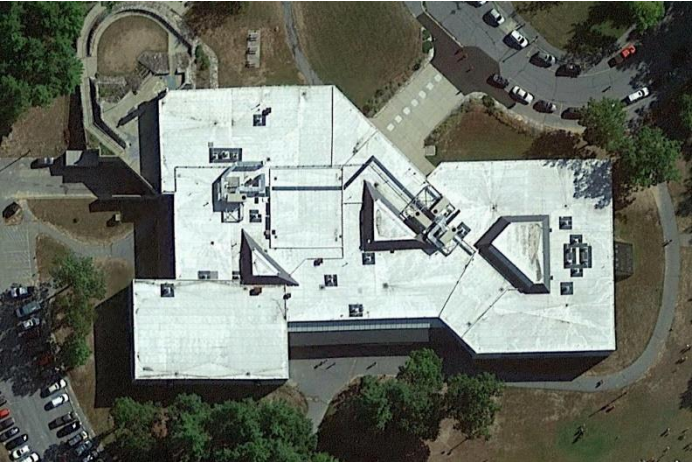
2.1 Aerial photo of the roof.
