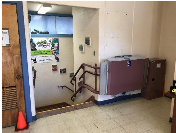
3.25 Handrail on lobby stair to cafeteria
