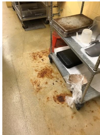
3.25 Kitchen epoxy floor.
