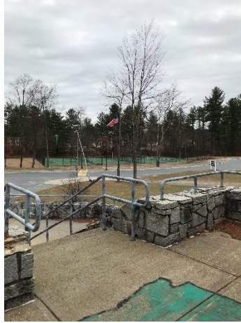
1.8 Handrails at concrete patio play area.
