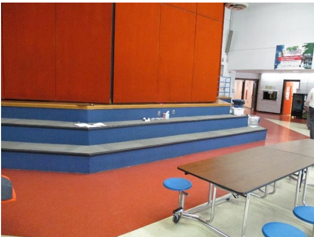
3.24 Sheet vinyl floor at cafetorium.
