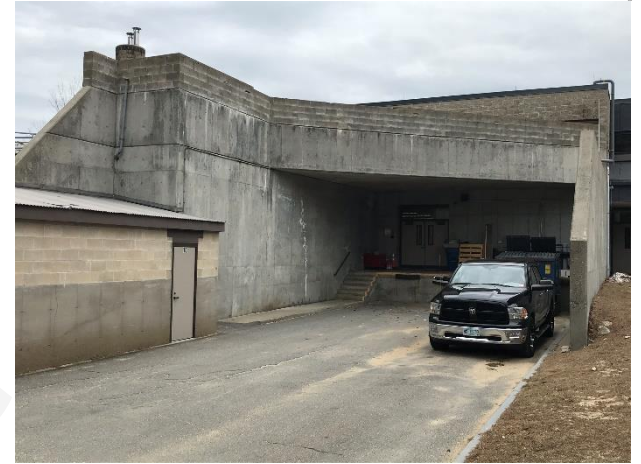
1.9 CMU wall at concrete patio and loading dock area.
