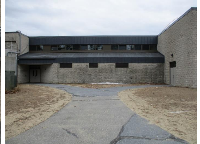
2.3 Sloped roof by the loading dock area.
