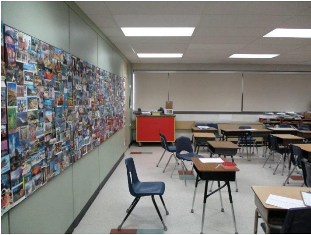
3.1 Demountable partition between classrooms.
