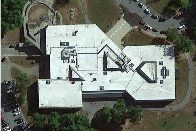
2.1 Aerial photo of the roof.
