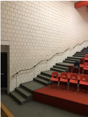
3.30 Handrail in the auditorium.
