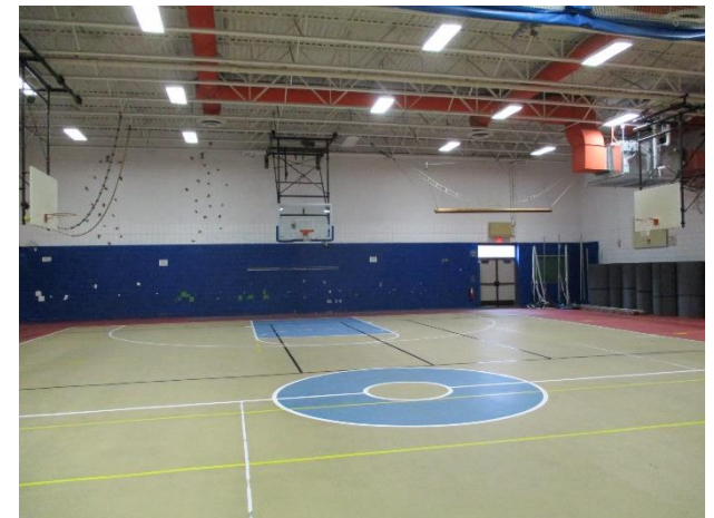
3.26 Gymnasium floor, walls and ceiling.
