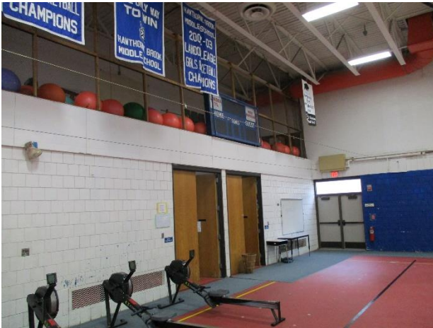
3.27 Gymnasium storage area.
