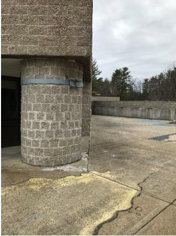
1.7 Concrete patio play area.
