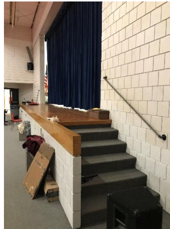
3.31 Handrail to the stage.
