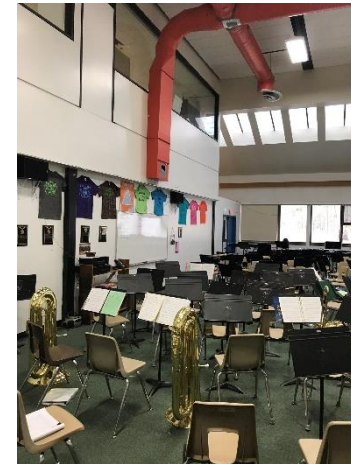
3.7 Skylight at Band Room.
