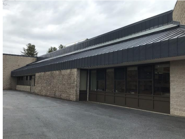
2.2 Sloped roof by the Music Room.
