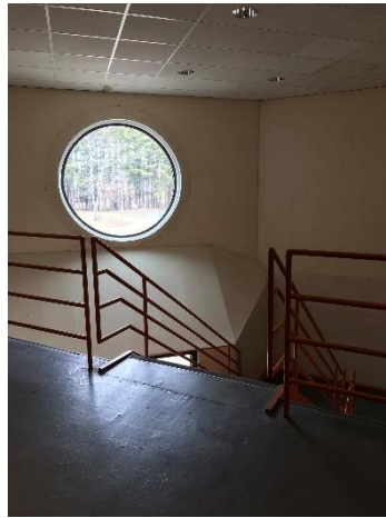
3.34 Handrails at Stair B.
