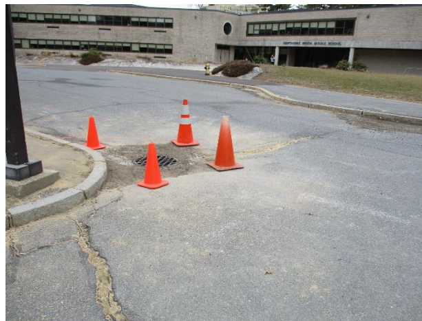
1.5 Newly replaced catch basin.
