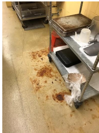
3.25 Kitchen epoxy floor.
