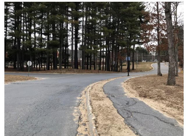
1.6 Granite curbs at bus drop off area.
