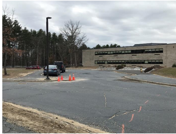
1.2 Bituminous paving at bus drop off.
