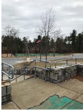
1.8 Handrails at concrete patio play area.
