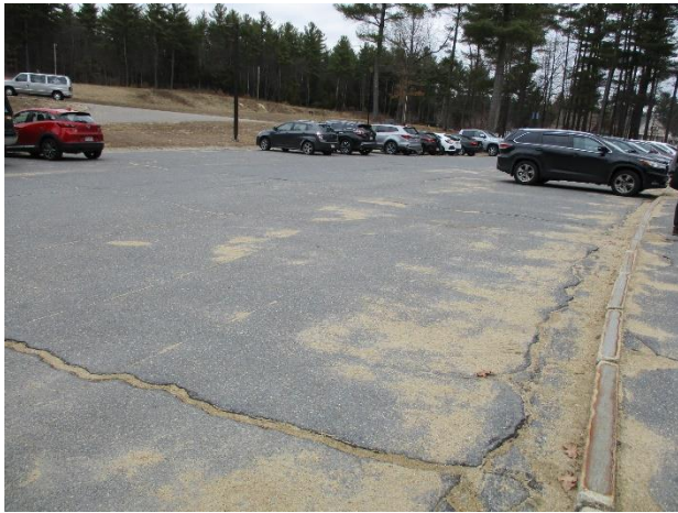
1.1 Bituminous paving at parking lot.
