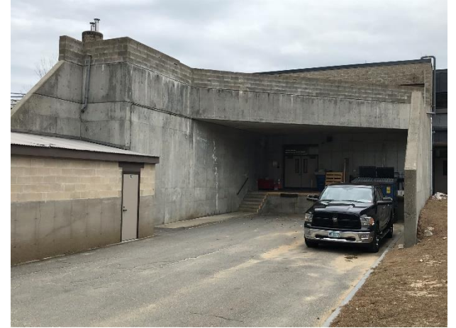
1.9 CMU wall at concrete patio and loading dock area.
