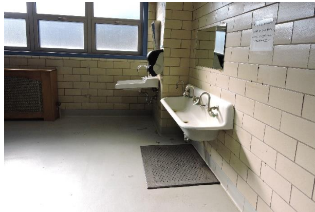
3.9 Toilet rooms in the 1950 building
