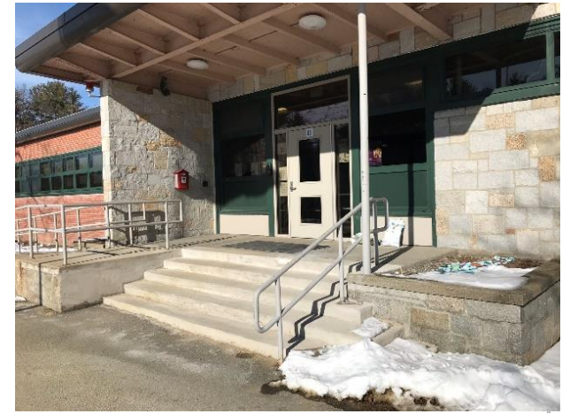
1.6 Canopy at main entrance
