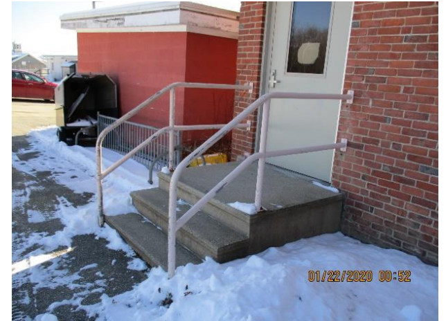
3.22 Gym egress stair
