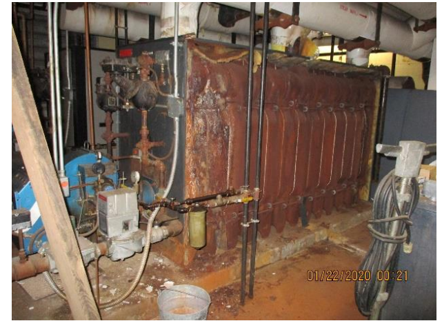
4.7 Non-functioning boiler
