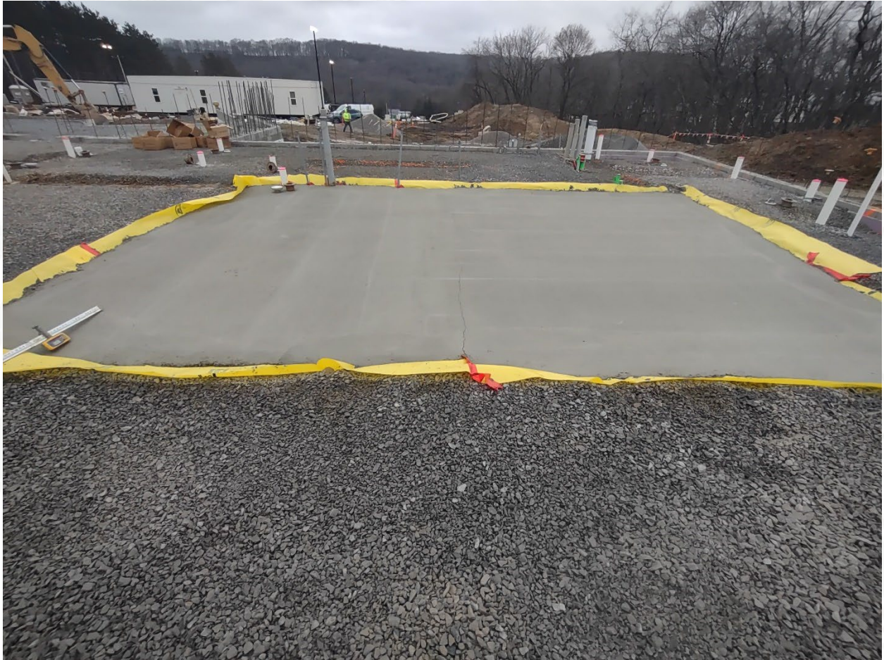
Depressed slab elevation for new Walk-in Refrigerator and Freezer This area is visible in cover page image.
