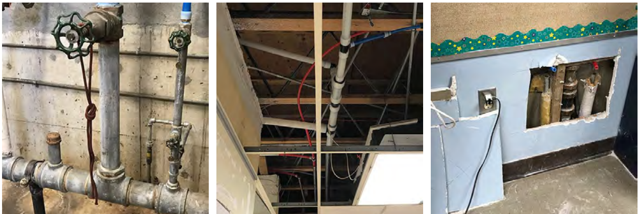
Aug. 19 - domestic water pipe replacement
