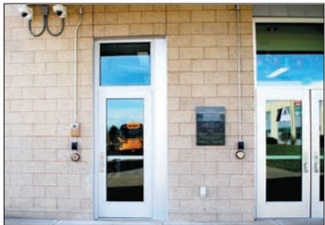
▲ At Quatama, a new door was carved out of the building to create a new entry vestibule into the main office.
