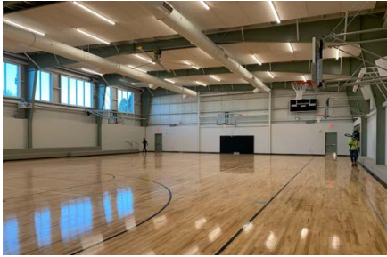
New gymnasium at Mooberry Elementary
