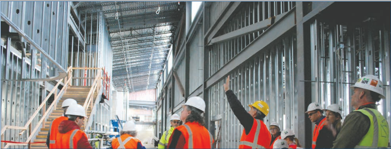
▲Tamarack ES: the Citizens' Bond Oversight Committee, comprising community volunteers, views the building's progress in just one of many visits they have made over several years of bond construction.
