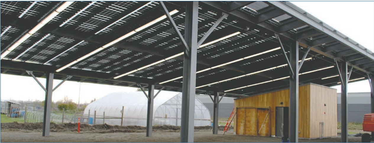
▲Liberty HS: the solar array canopy was substantially completed in early April, and will provide hands-on experience with solar power generation for students learning about sustainable technologies and design
