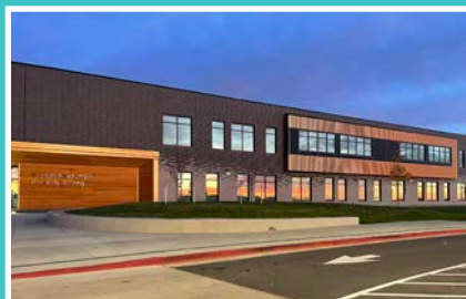
Tointon Academy of Pre-Engineering
