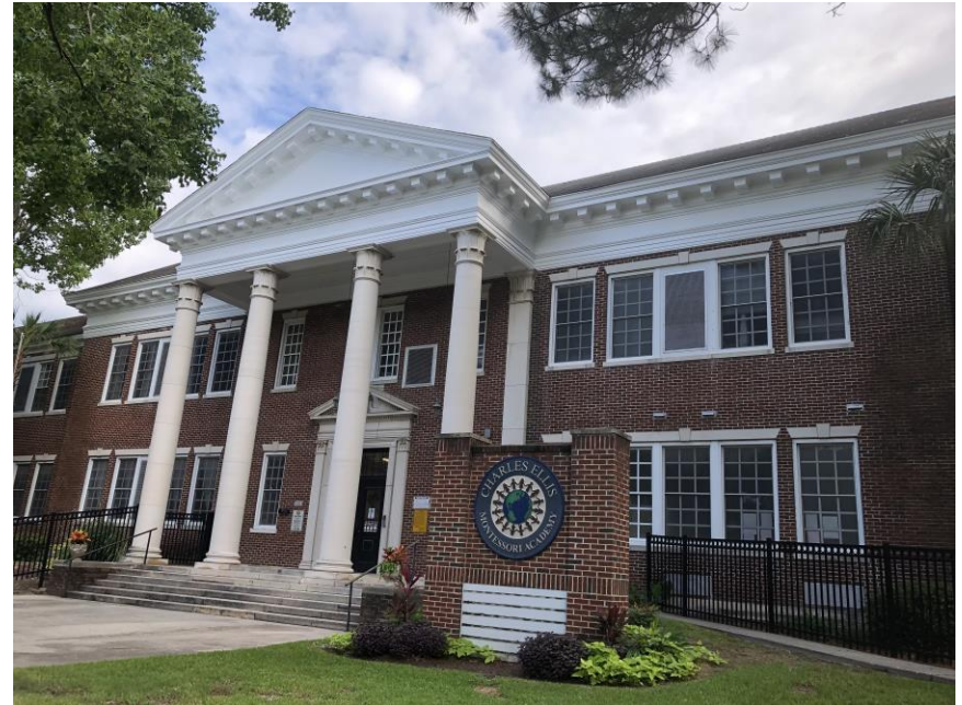
Completed portico at the Charles Ellis Montessori Academy K8
