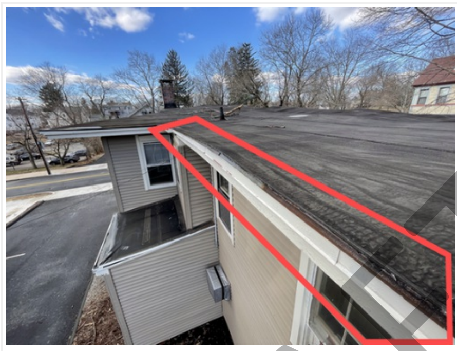
Photo 15 Open condition- Perimeter edge lifting
