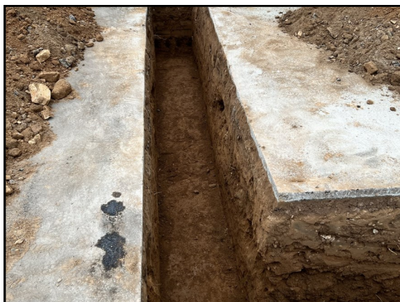
Altadena trench for new fire hydrant
