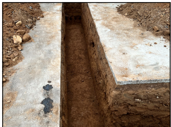
Altadena trench for new fire hydrant
