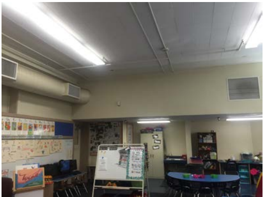
Building A Typical classroom air distribution with above ceiling fan coil
