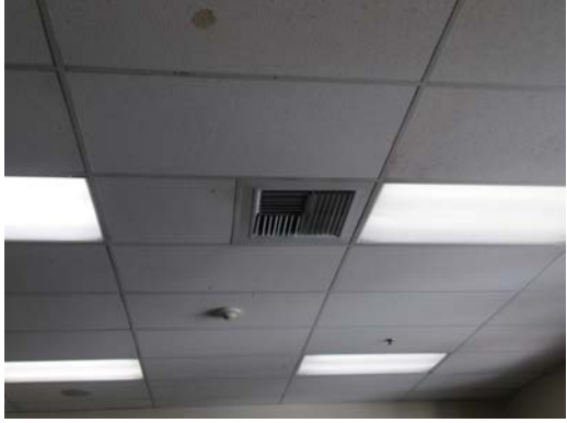
Building D – Room 106 Diffuser filter requires maintenance
