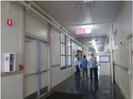
Building A – Room 115 ADA violation – 4 in. max protrusion for fire extinguisher
