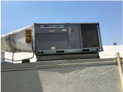
Building A – Exterior Auditorium rooftop mounted AC unit within 10 feet of roof edge
