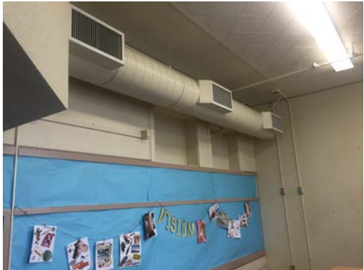
Building A – Typical supply air ductwork
