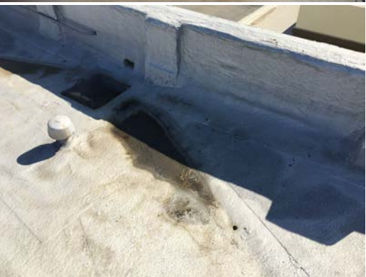
Building A – Roof Water accumulation
