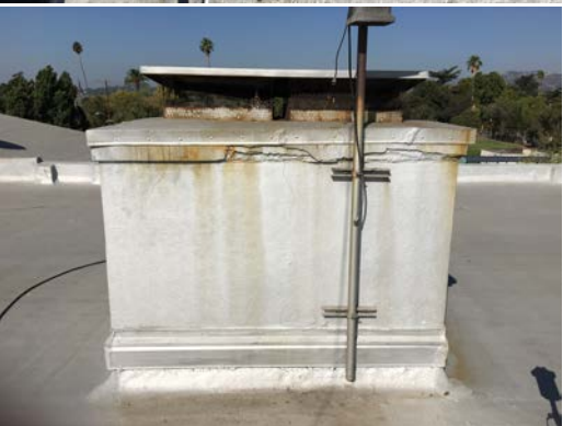
Building A – Roof Vent damaged
