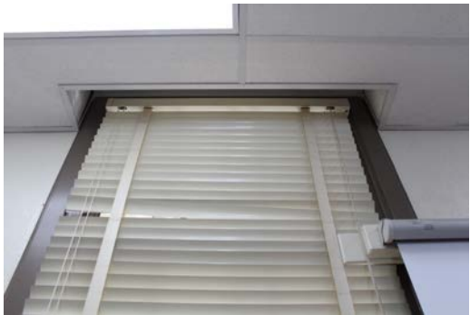
Building A – Room 128 Window cutting through A/V and ceiling
