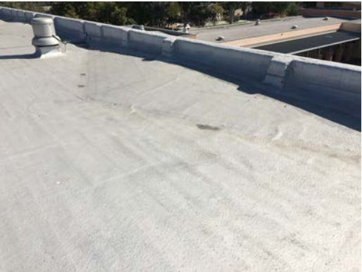
Building A – Roof Bubbling
