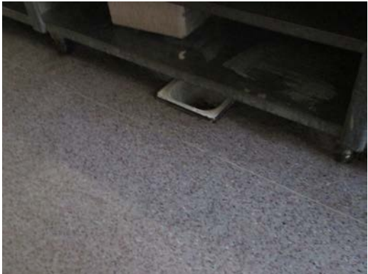
Building B – Room 101 Floor drain unused
