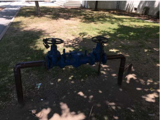
Exterior – Reduced pressure backflow preventer
