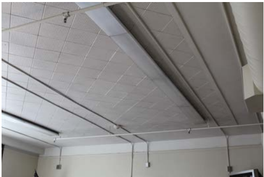
Building A – Room 106 Sprinkler/lighting overlapping
