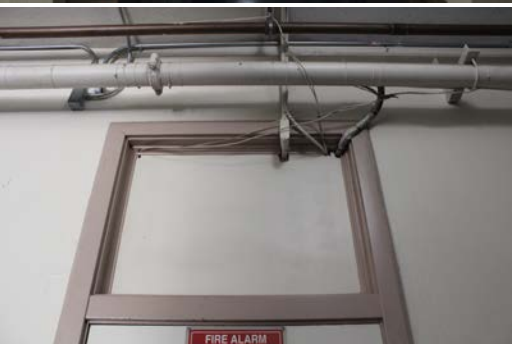
Building A – Room 115 Exposed wire pipe
