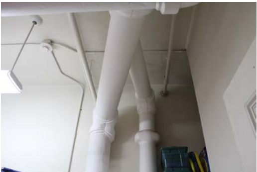
Building A – Room 112 Crisscrossing pipes Relocate per mechanical
