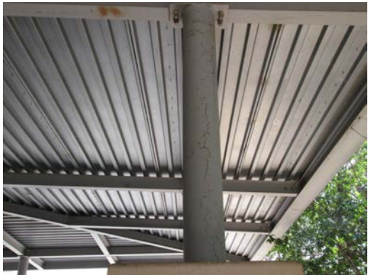
Building D - Exterior Column/decking damage
