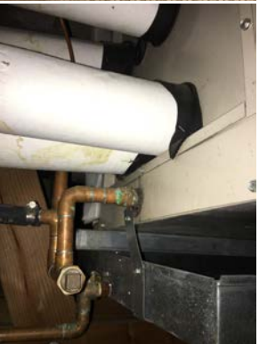
Building A – Leaking ceiling at 1 st floor due to issues with saw cut restroom on second floor above
