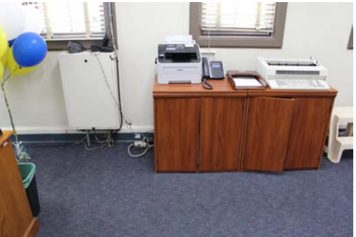
Building A – Room 120 Electrical panel exposed
