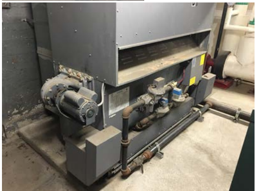
Building A – B01 Failing boiler
