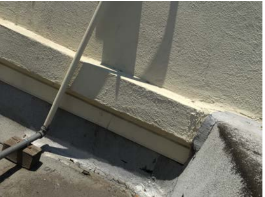
Building A – Auditorium Rooftop mounted gas piping sleeper attached with mastic
