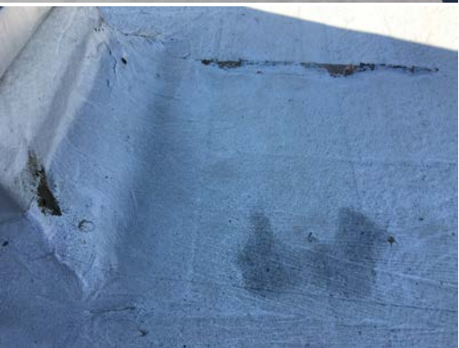
Building A – Roof Bubbling
