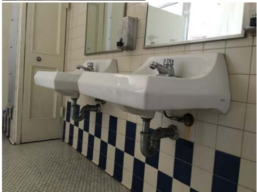
Building A – Room 201 Missing insulation on fixtures
