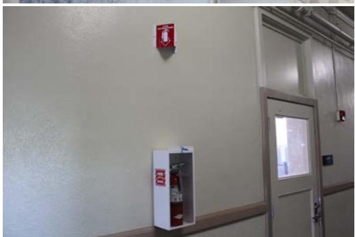
Building A – Room 212 ADA violation – 4 in. max protrusion fire extinguisher
