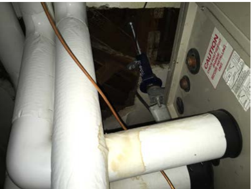
Building A – Typical above ceiling 4-pipe fan coil installation with vibration isolation
