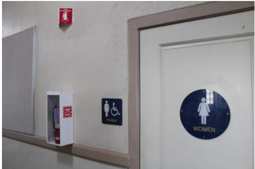
Building A – Room 115 ADA violation – 4 in. max protrusion for fire extinguisher
