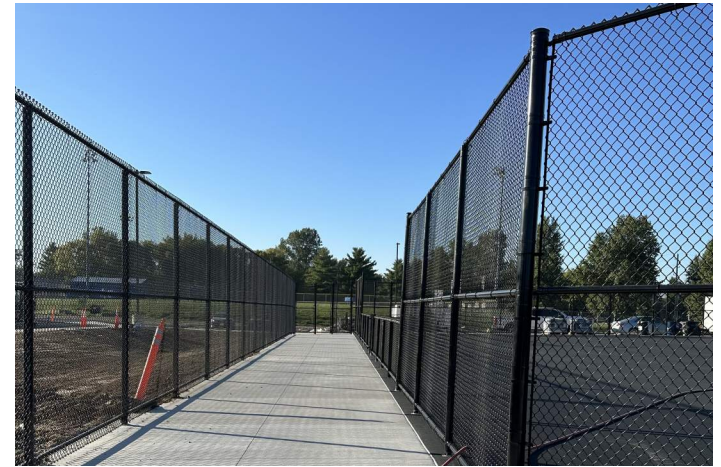
East Concourse Looking South
