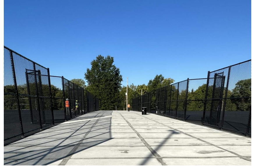
Center Spectator Area Surfacing Prep - Looking West
