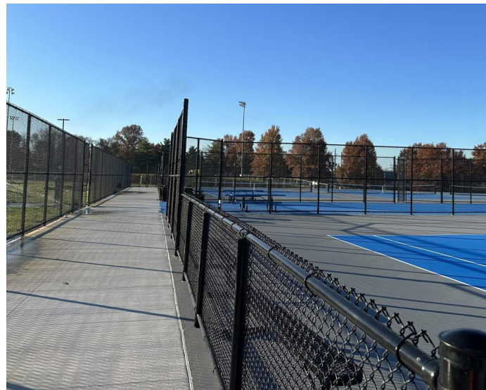
East Concourse Looking South
