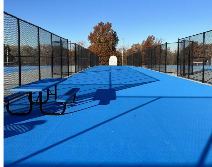
Center Spectator Concourse Looking West
