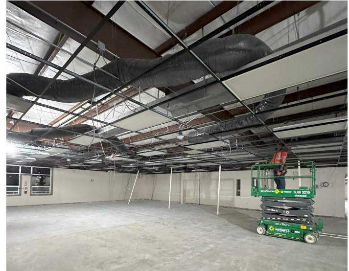
District Technology Center
