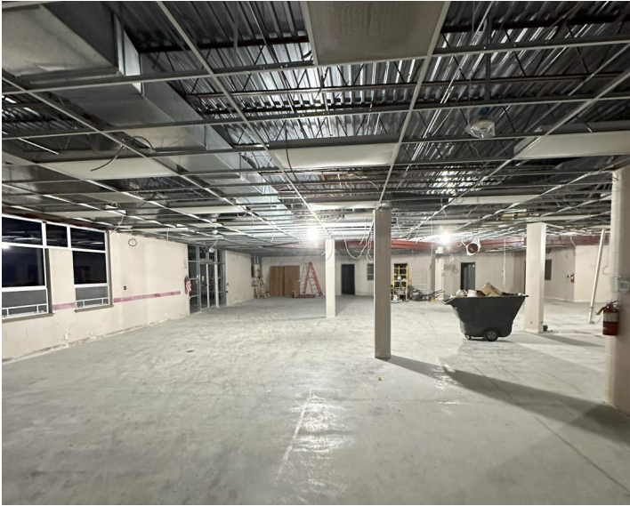
District Technology Center
