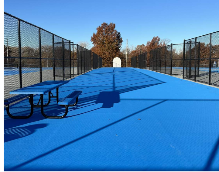
Center Spectator Concourse Looking West
