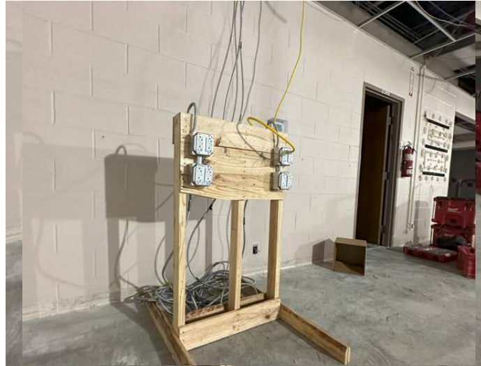
District Technology Center
