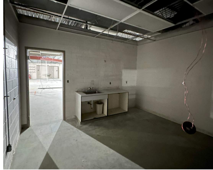
District Technology Center
