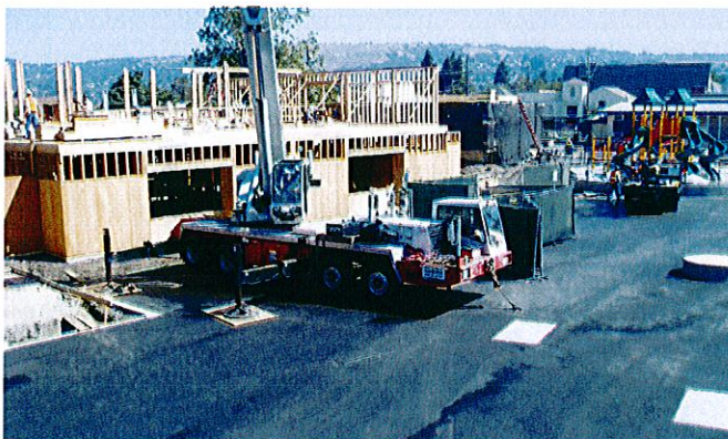
Construction of New Two-Story Classroom Building at Highland Elementary School
