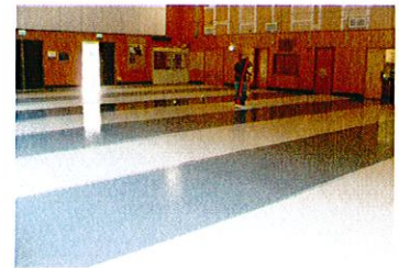
New Floor for Renovated Multi-Purpose Room at Montera Middle School
