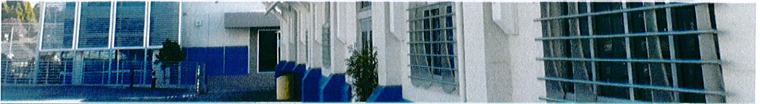
Renovated Classroom Building with New Canopy at Oakland High School
