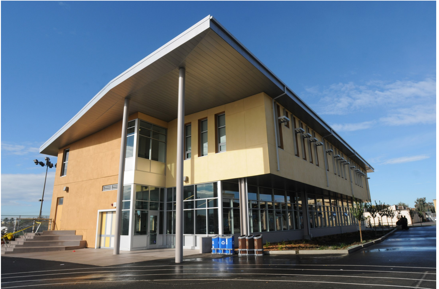
Coliseum College Prep Academy and Roots International Academy at Havenscourt New Classroom & Cafeteria Building
