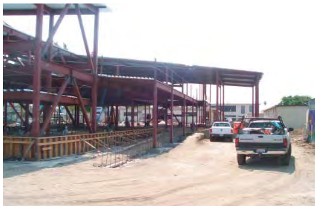
Cox Elementary - Framing for New Building
