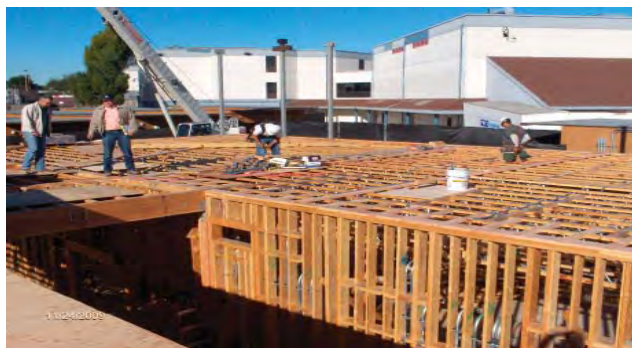
Oakland High School - Framing for New Building
