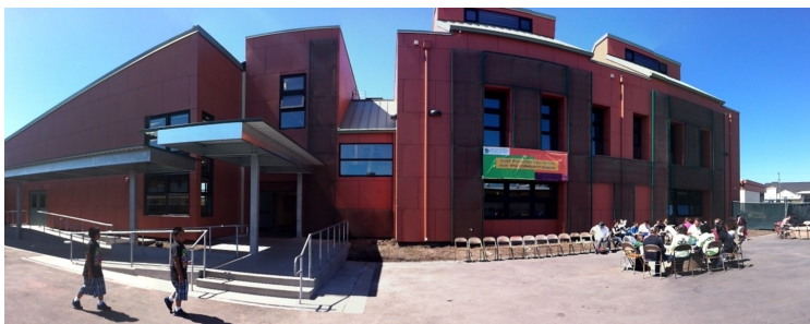
Highland ES New Classroom & Cafeteria Building
