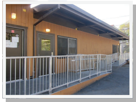
Existing Claremont Interim Kitchen
