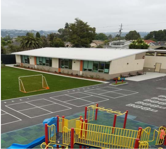
Greenleaf at Whittier - New construction K-2 Modular Classroom Building, Field and Play Area
