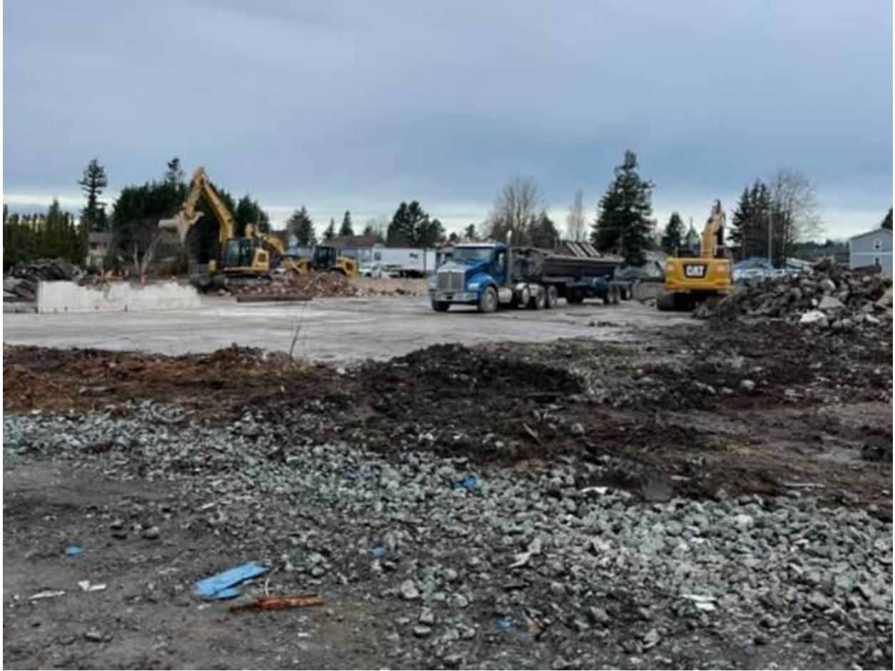
The last bits of debris being hauled off-site
