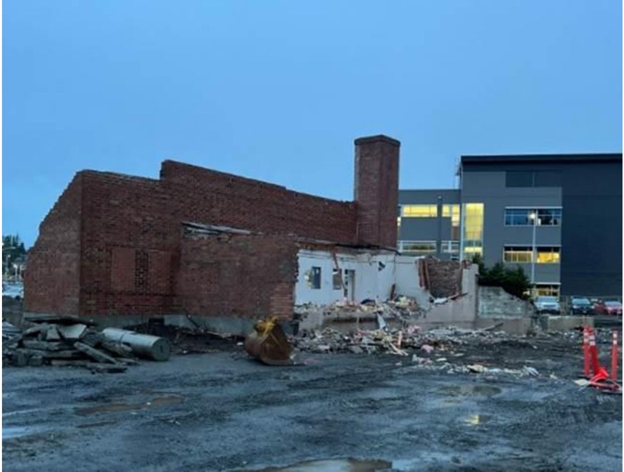
The last piece of Old Main that was demolished this week
