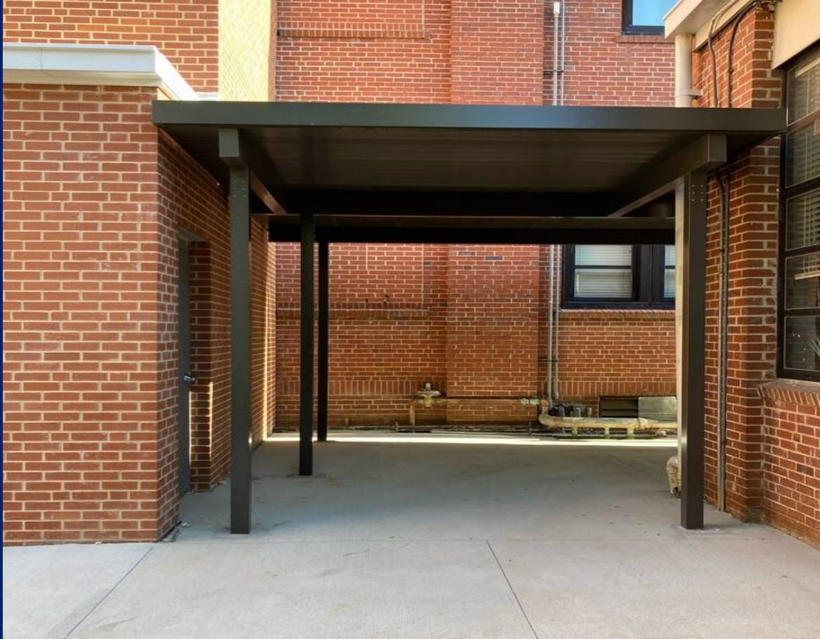
Awning at new elevator
