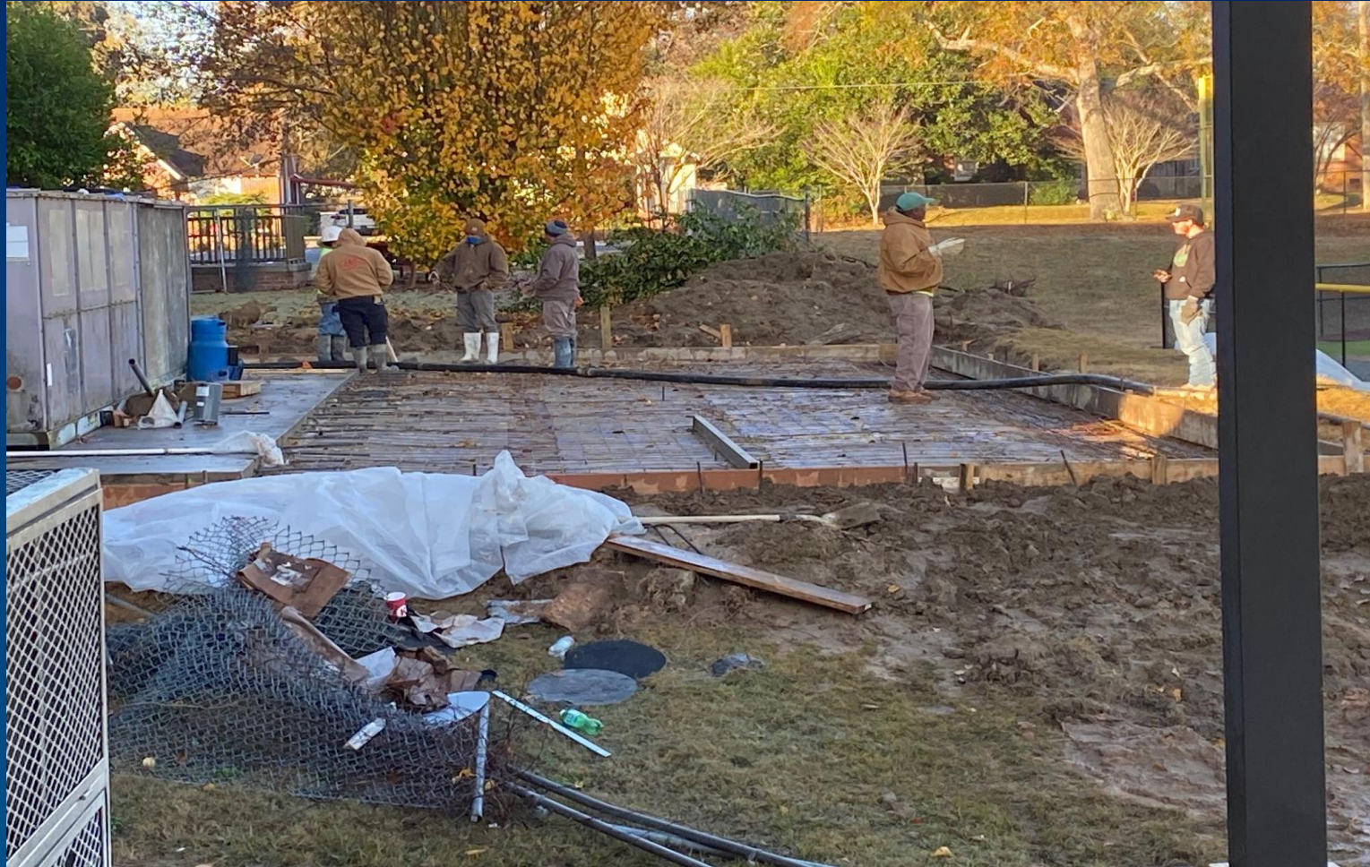
Foundation to Support New HVAC Equipment
