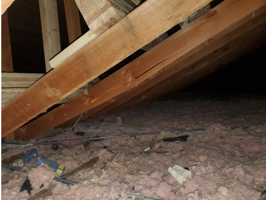
1913 Building: Failed Roof Joist at Overbuild
