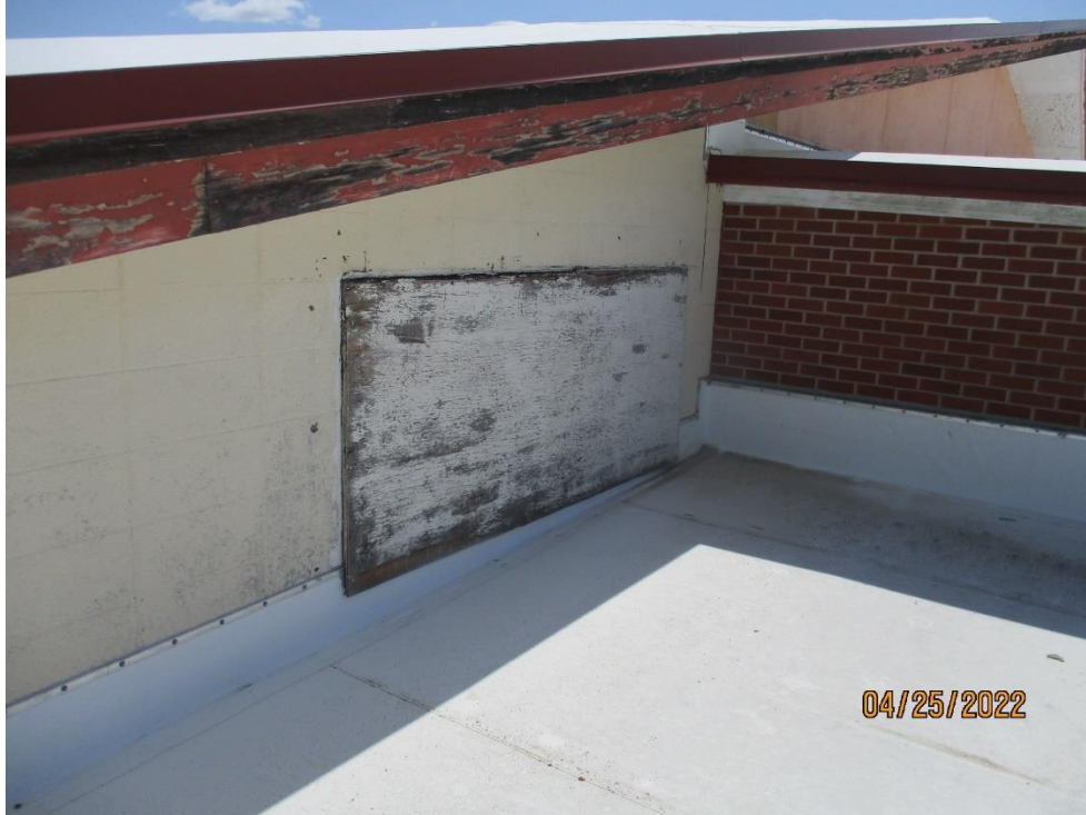
1967 Building Roof Area B: Plywood attached to the gym wall. Deteriorated and not water tight.
