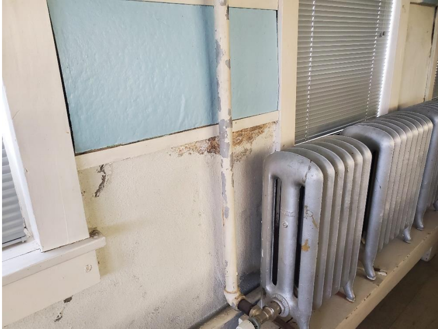
1913 Building: Foundation Deterioration At Interior Face of Wall
