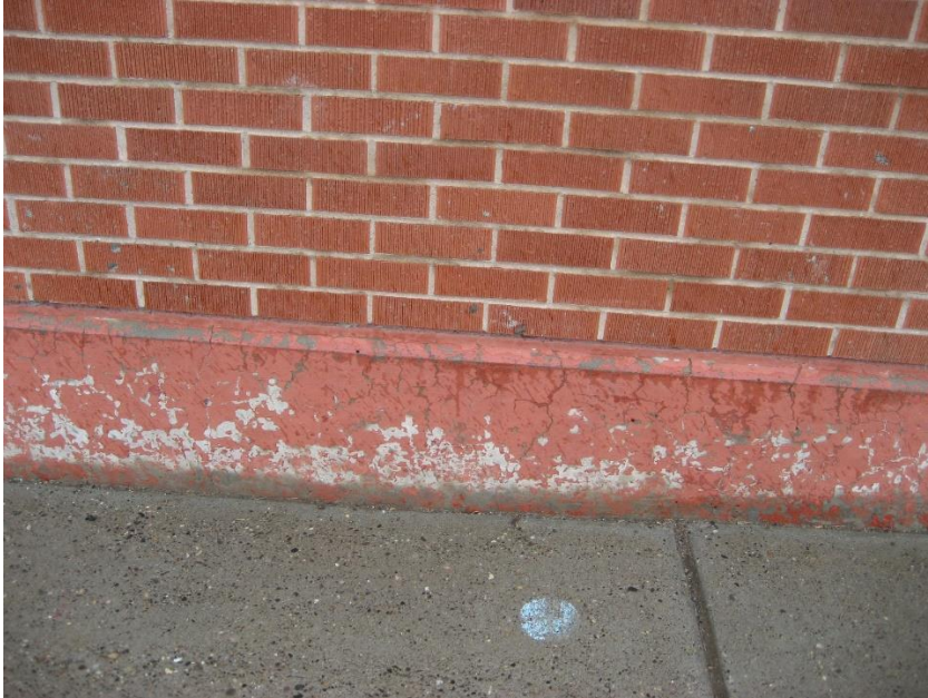
Figure 11 – Chipped and peeling paint at foundation wall.
