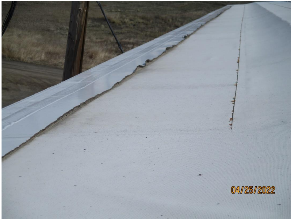
1967 Building Roof Area D: Strip in edge is failing on the gym.
