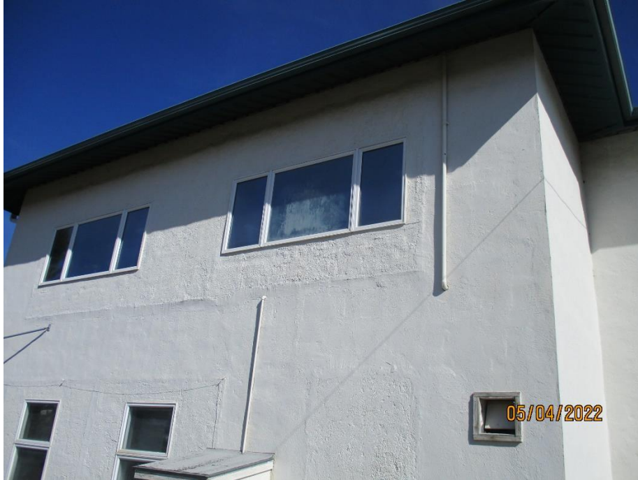
1913 Building: Window seal has failed.
