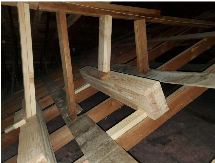
1913 Building: Prior Repair at Failed Roof Joist
