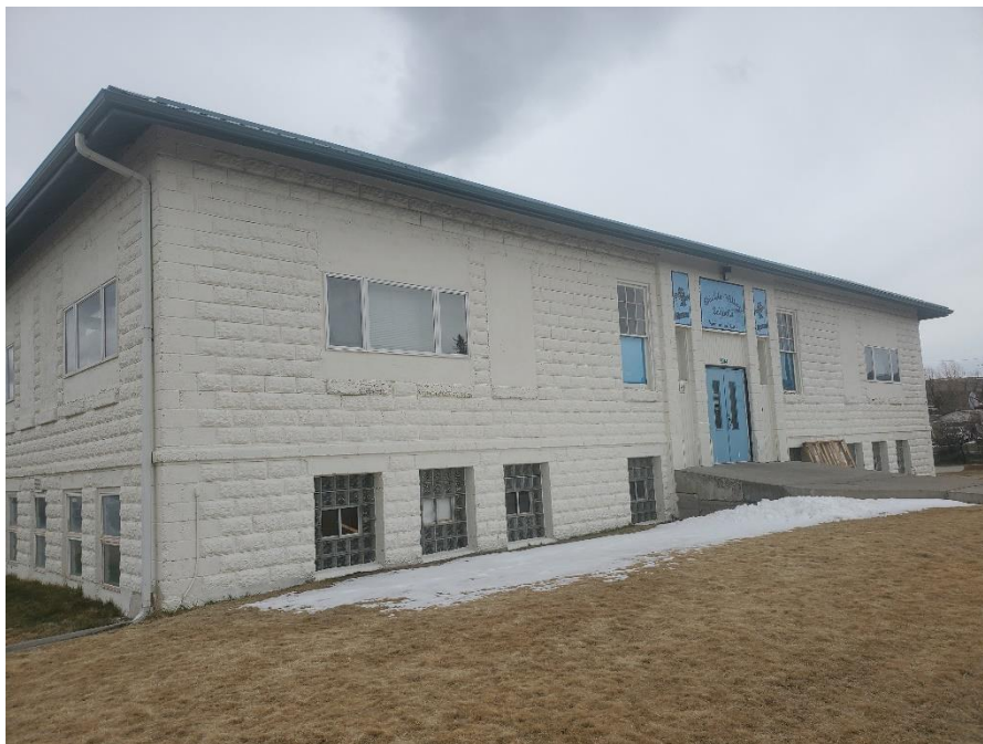
1913 Building: Adverse Grades at North Side of Building
