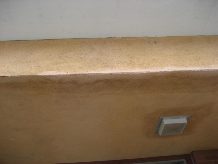
Figure 13 – Patched stucco soffit at ceiling of Main Entry.
