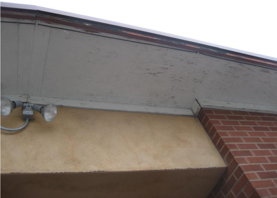
Figure 14 – Peeling paint typical at wood soffit and fascia at perimeter of building.
