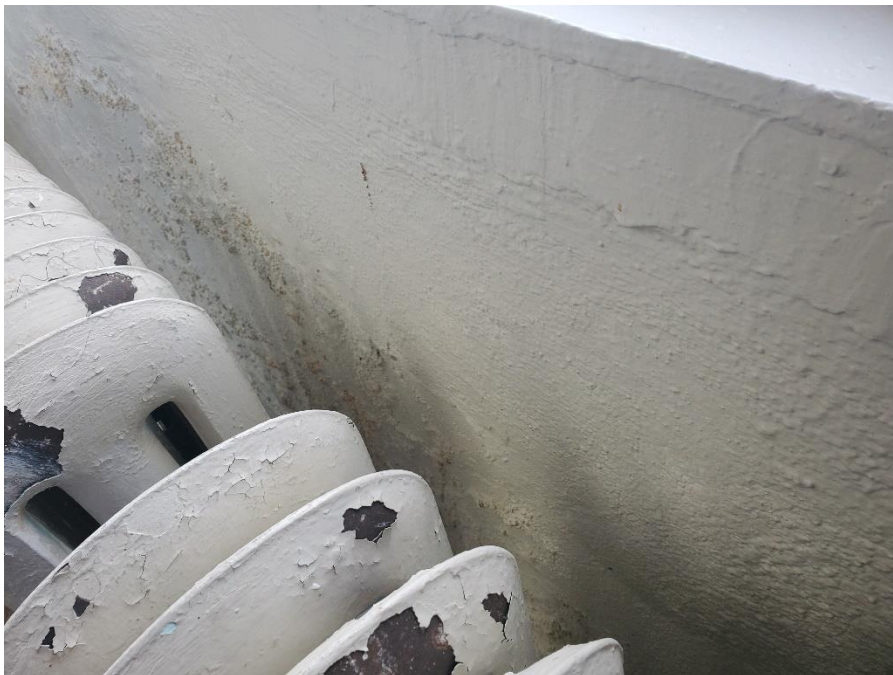
1913 Building: Foundation Deterioration at Interior Face of Foundation
