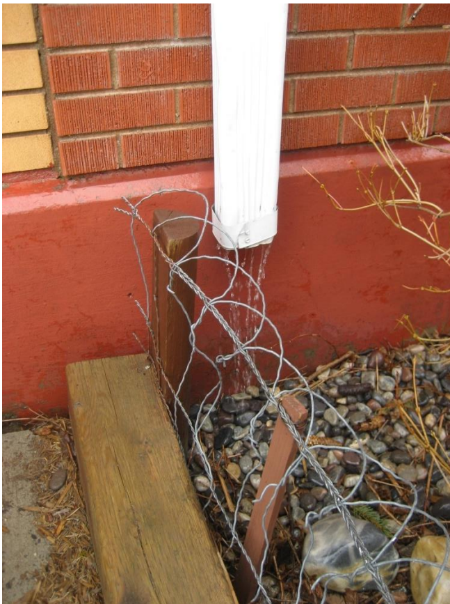
Figure 12 – Downspout missing rain leader at foundation wall.
