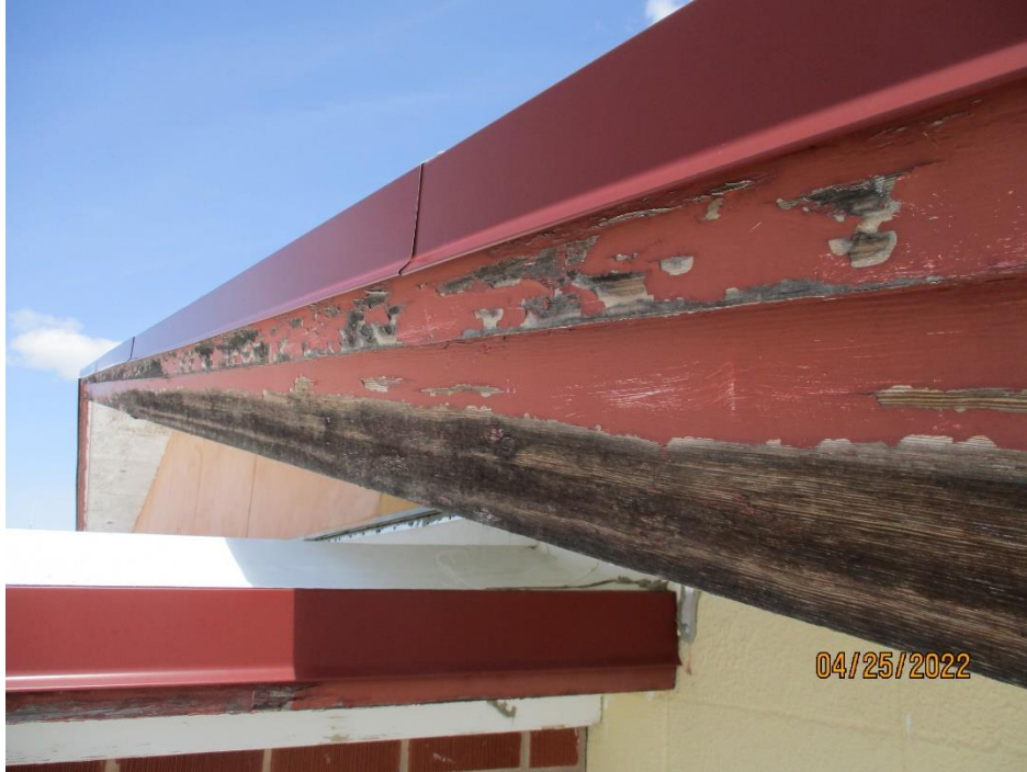
1967 Building Roof Area D: Fascia wood face should be clad with metal.
