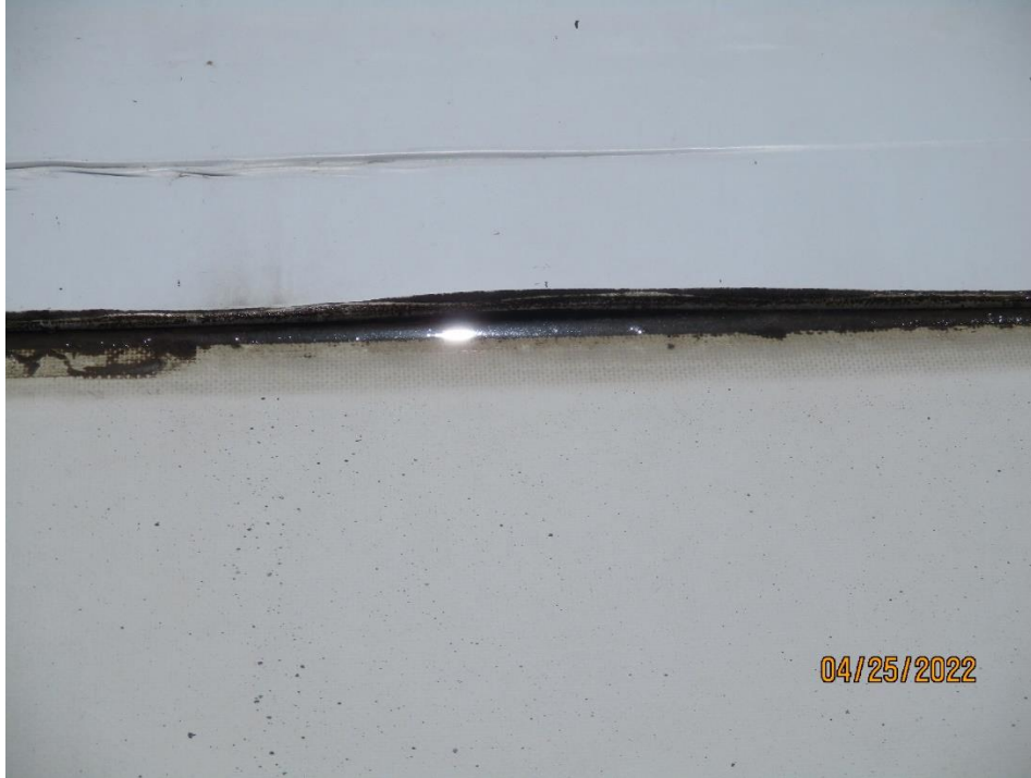
1967 Building Roof Area D: Water is bucking at the strip in edge.
