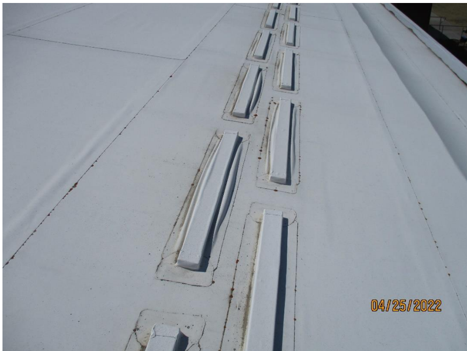
1967 Building Roof Area D: Wind uplift at snow retention.
