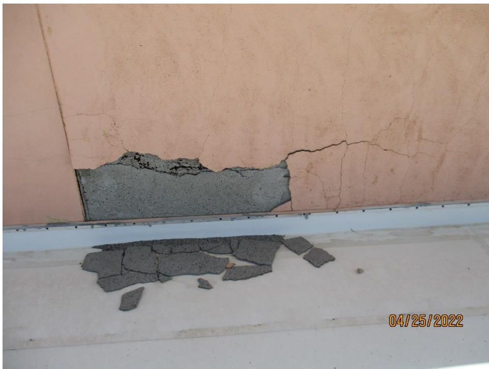
1967 Building Roof Area C: Entire stucco wall on the west side of the gym is failing.
