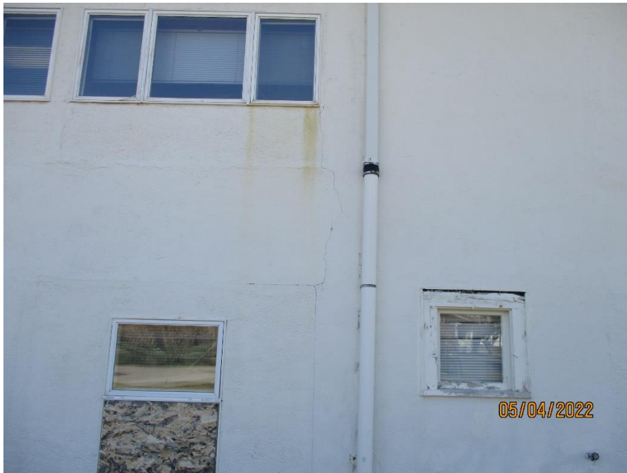
1913 Building: Cracks in stucco are evident as well as window frame has deteriorated.
