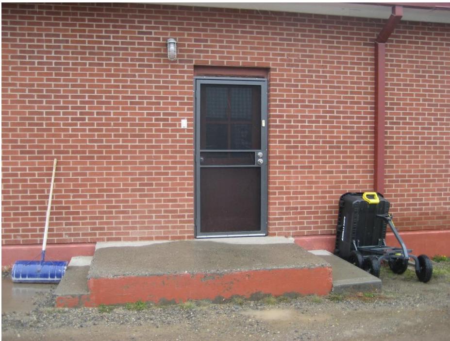
Figure 8 – Landing at exit door from Kitchen; missing guardrail.
