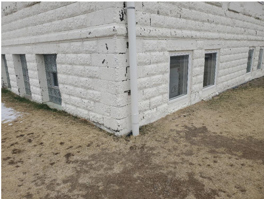
1913 Building: Adverse Grades and Foundation Deterioration at Northwest Corner of Building
