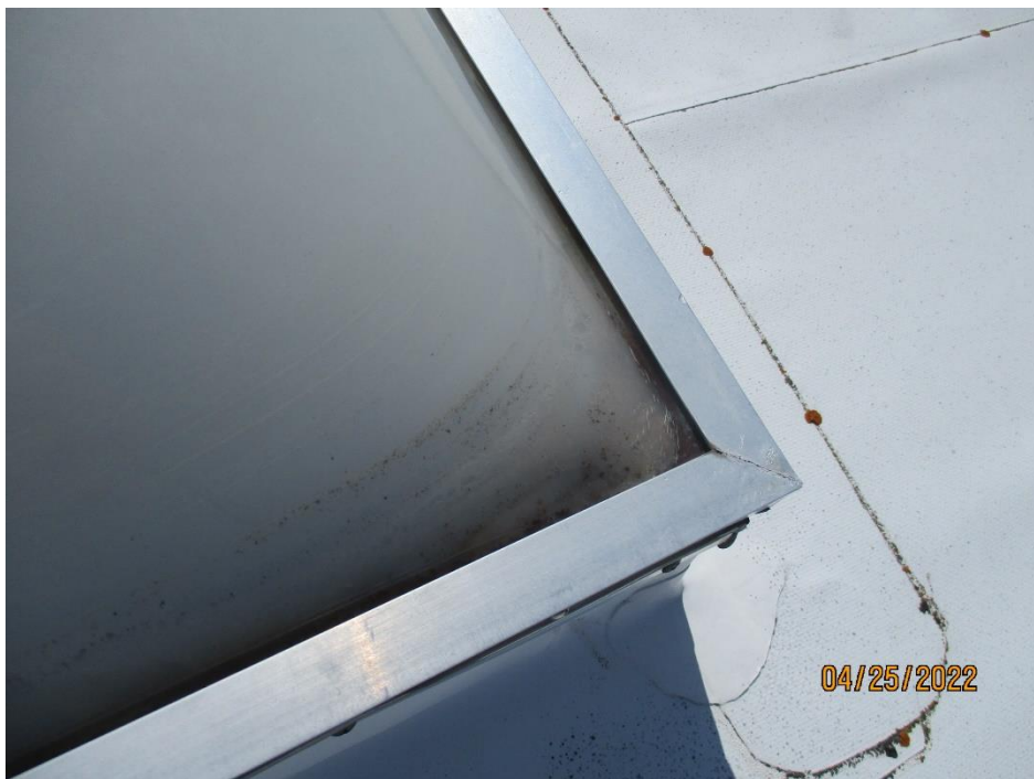
1967 Building Roof Area D: Skylight with moisture and cracking in corner.
