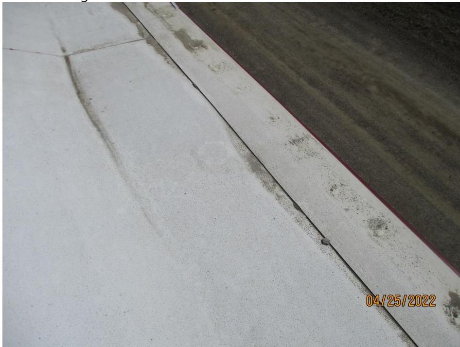
1967 Building Roof Area A: Edge Stripping
