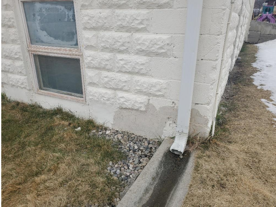
1913 Building: Adverse Grades and Foundation Deterioration at Northeast Corner of Building
