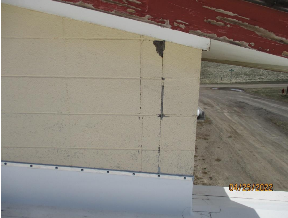
1967 Building Roof Area A: SW Corner of gym adjacent to roof section A is failing.
