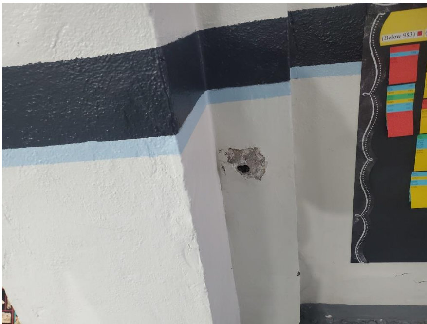
1913 Building: Alkali Silica Reaction on Interior Foundation Wall
