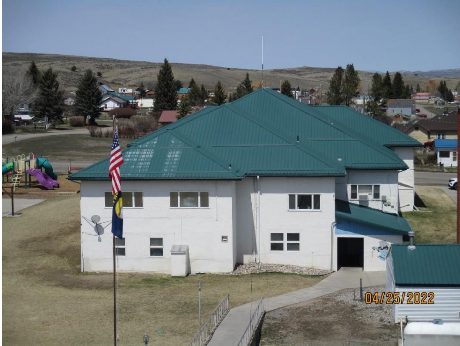
1913 Building: Metal panel paint is failing.
