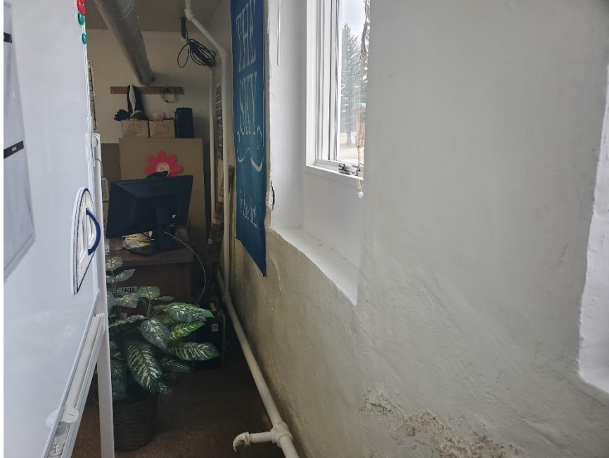
1913 Building: Foundation Deterioration at North Wall
