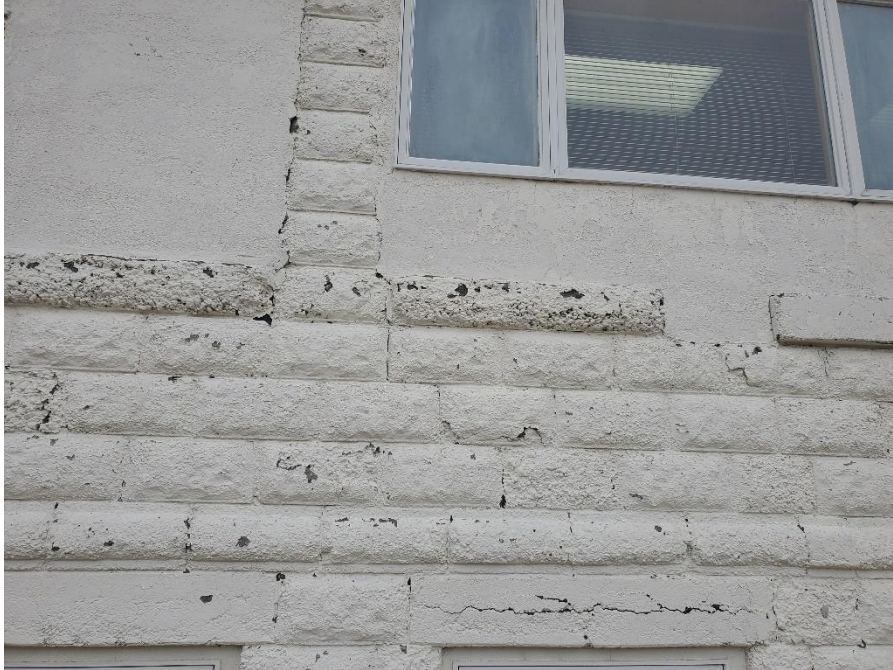
1913 Building: Masonry Deterioration Due to Moisture
