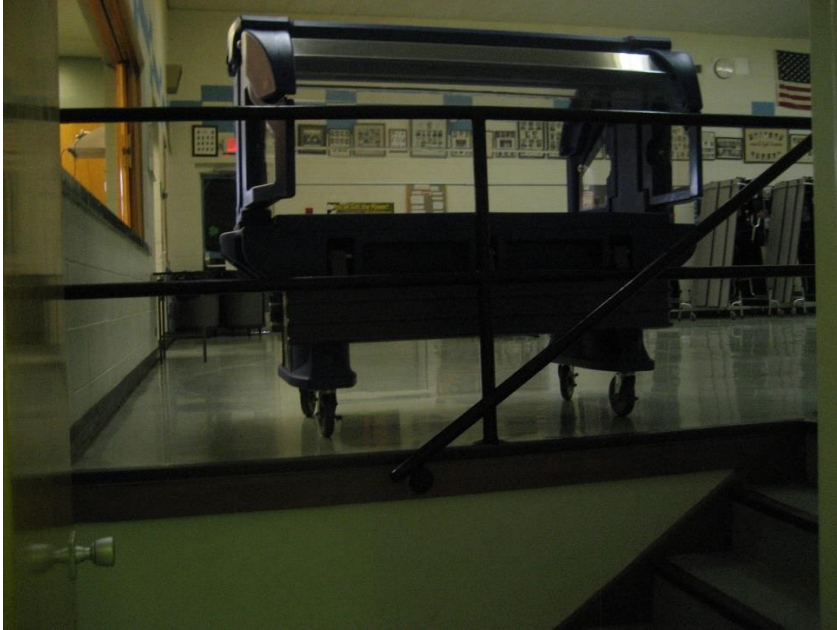
Figure 3 – Guardrail at Stair from Stage down to Gym level.
