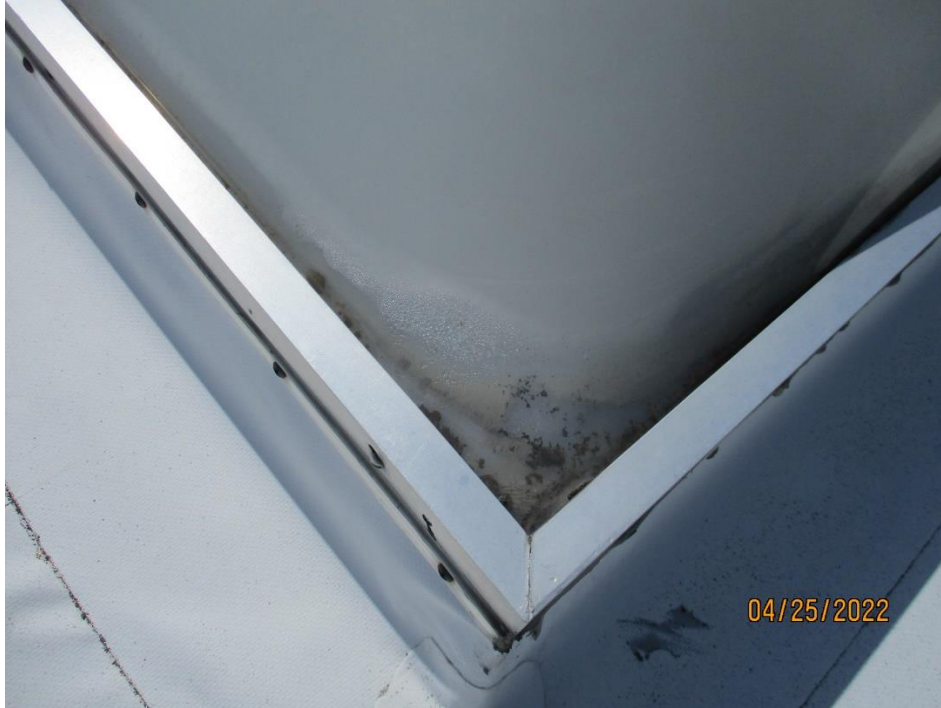
1967 Building Roof Area D: seals are broken. Moisture buildup in corner of skylight
