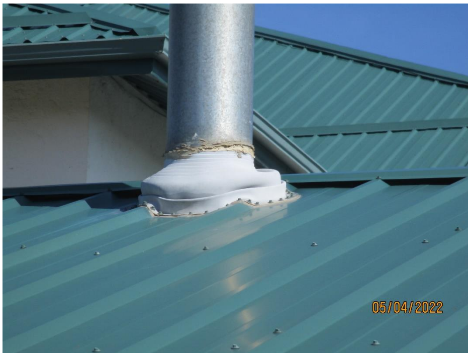
1913 Building: Pipe jack rubber gasket is failing.
