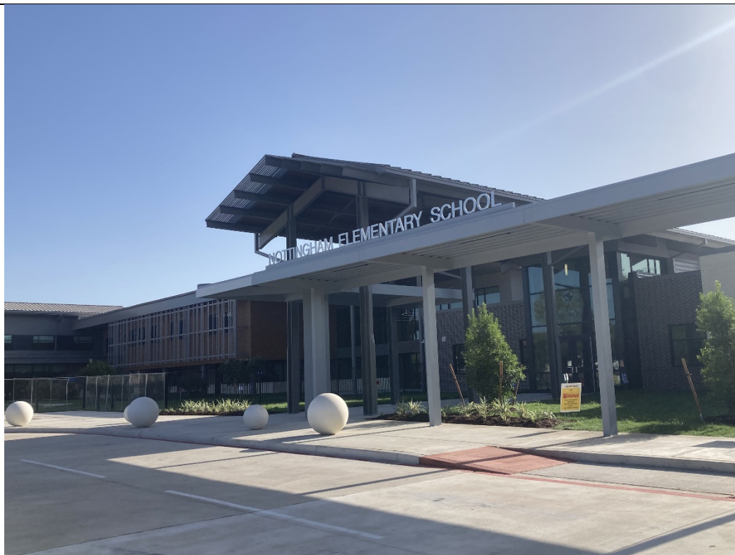
Exterior view at entrance canopy.
