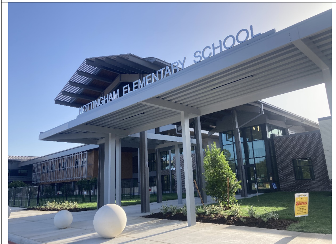
Exterior view at entrance canopy.
