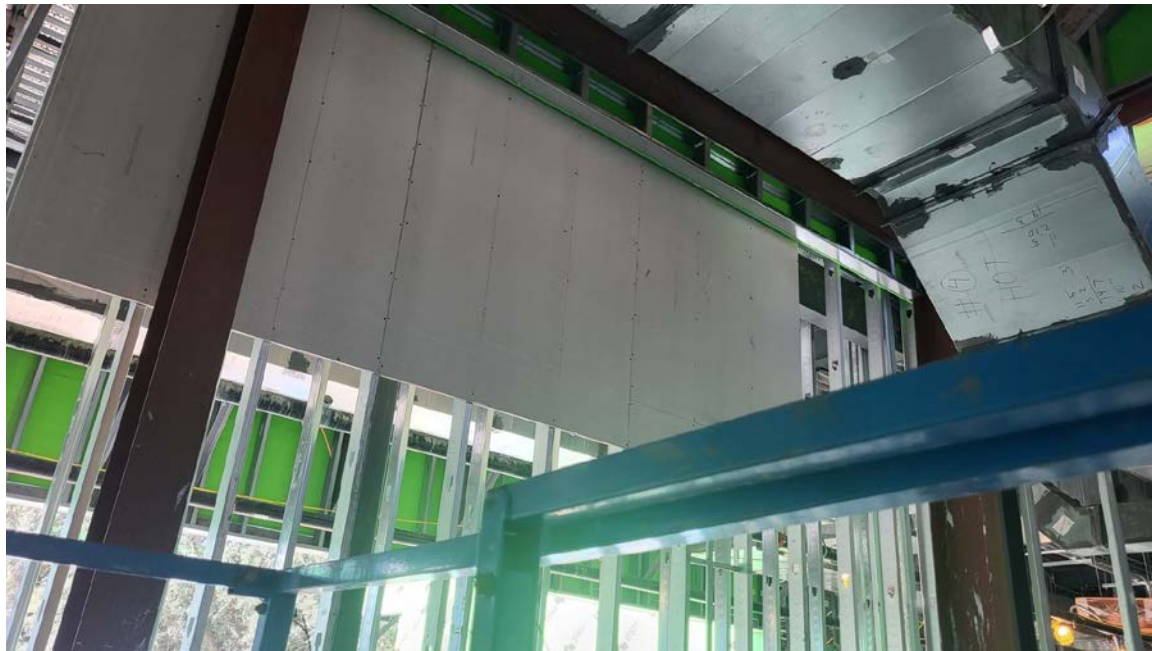
Above ceiling sheetrock install Area C
