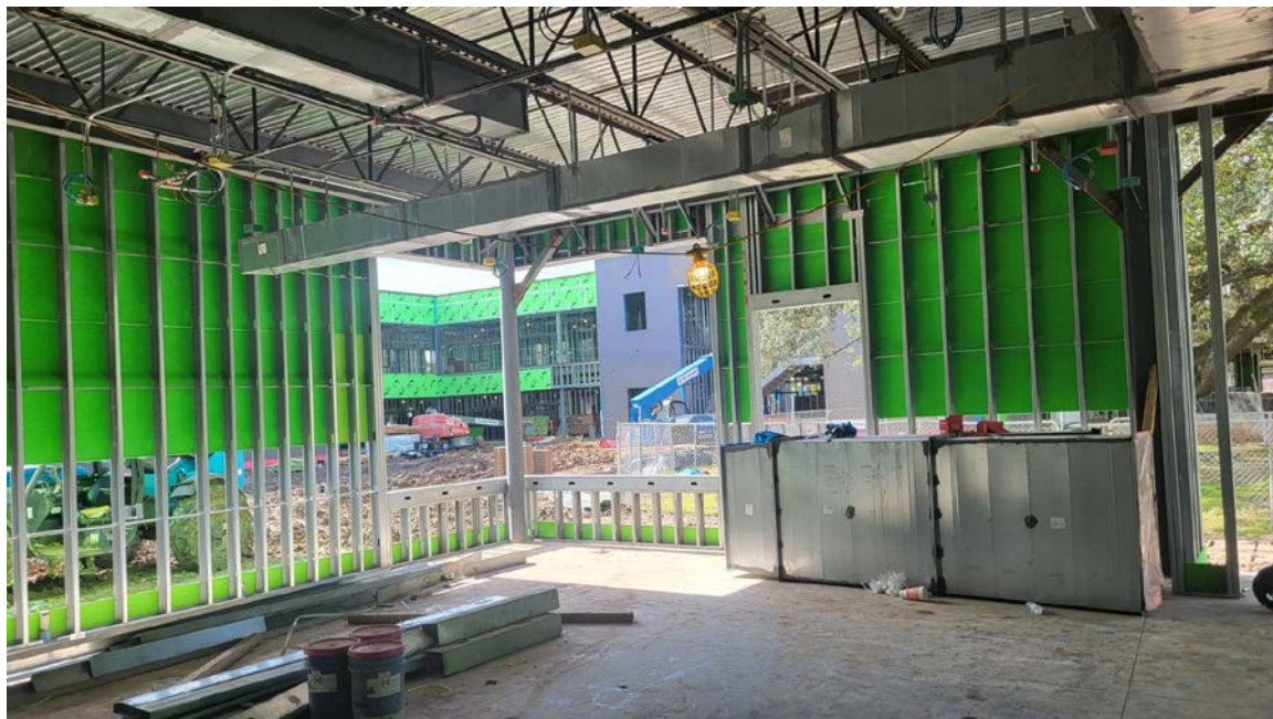
Exterior Wall Framing – Art Room interior
