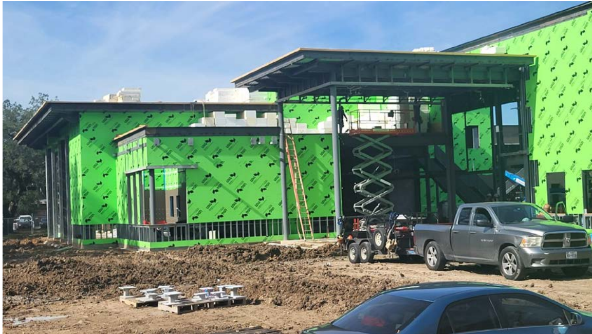
Area C Exterior Wall Sheathing
