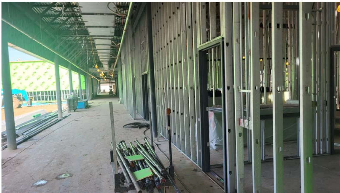
Area C Interior Wall Framing
