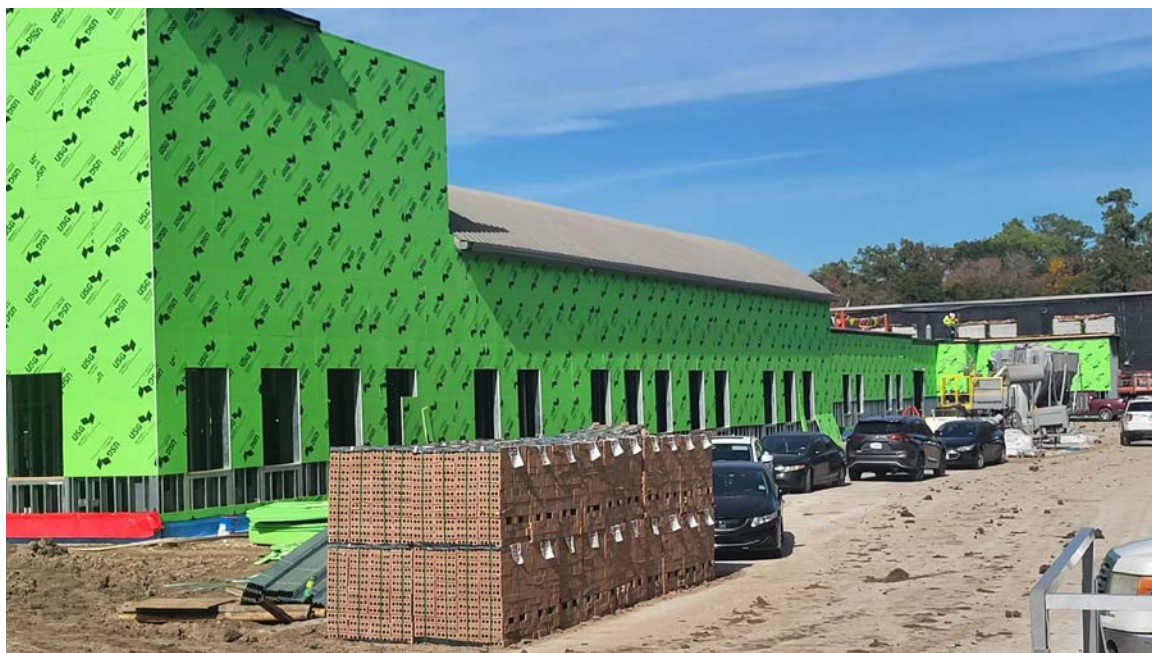
Area C Exterior Wall Sheathing
