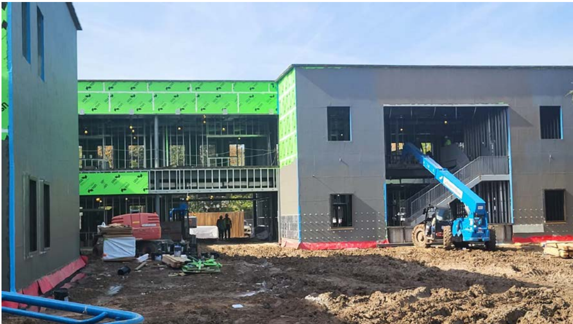
View of Area A/B corner in Courtyard
