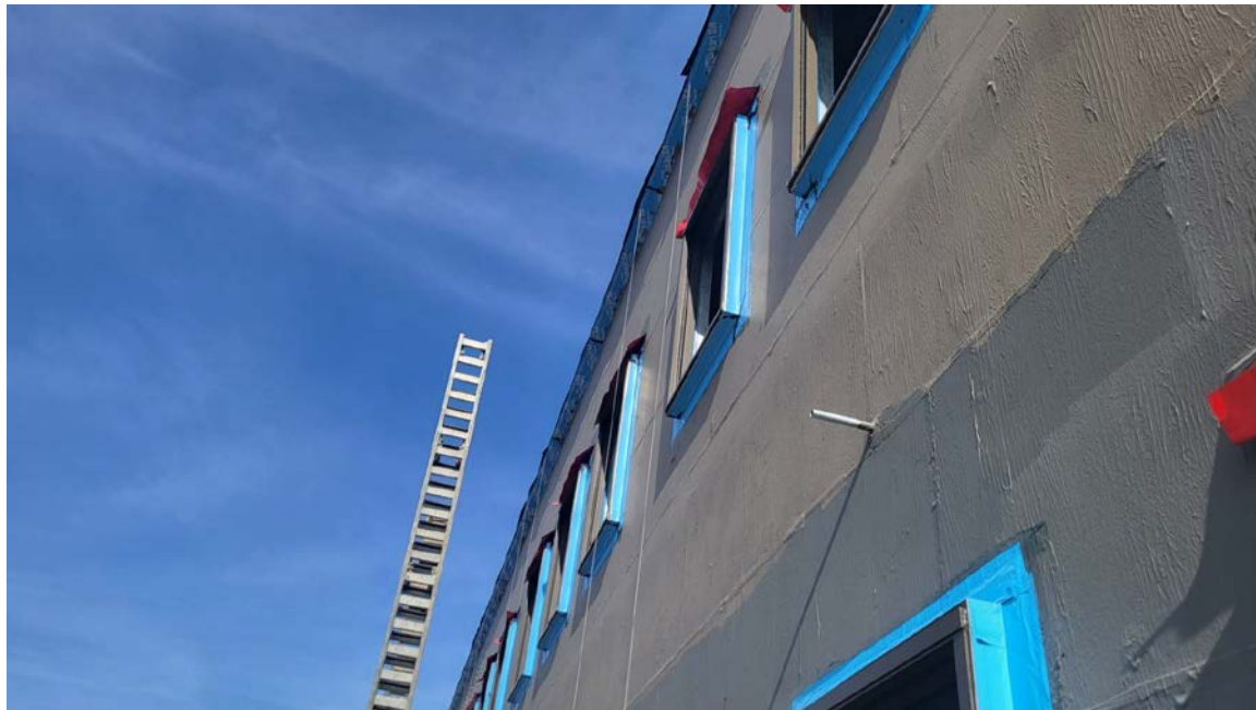
Exterior Window Frame Installation Area A
