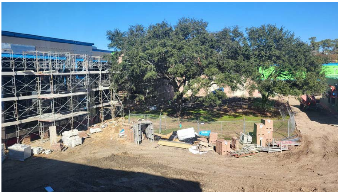
Courtyard View from 2 nd Floor
