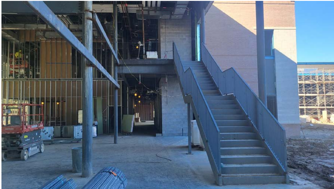
Stair Near Main Entry
