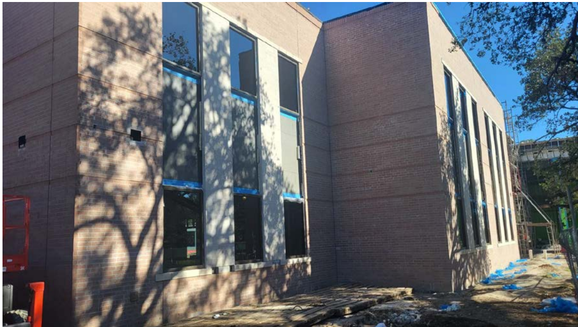
Masonry and Glazing Installed – Southwest Corner – Former Entry Location
