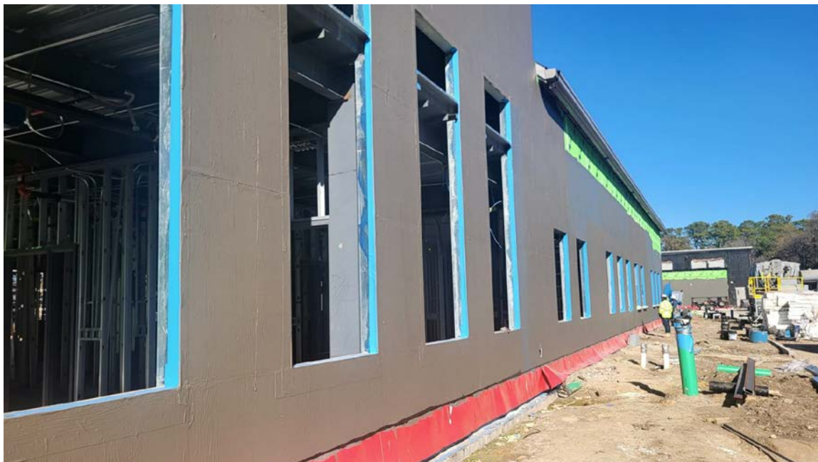
Area C East Elevation Waterproofing
