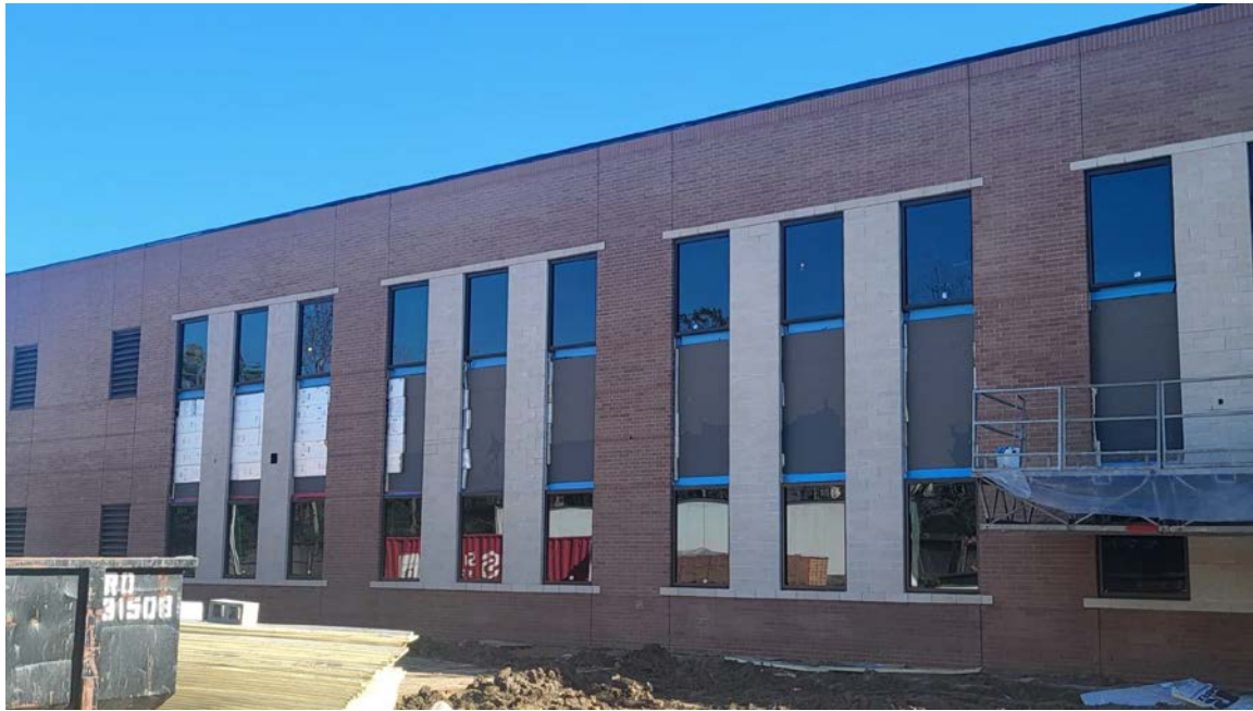
Masonry and Glazing Installed – West Elevation
