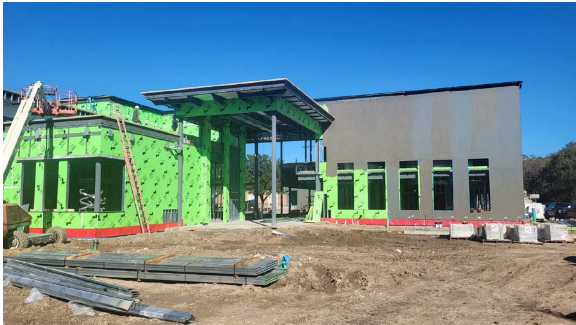
Area C East Elevation Waterproofing
