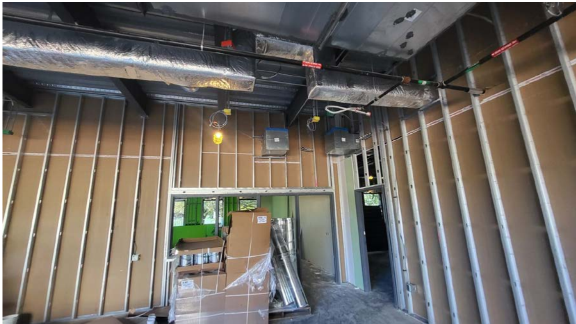
Classroom Sheetrock One Sided
