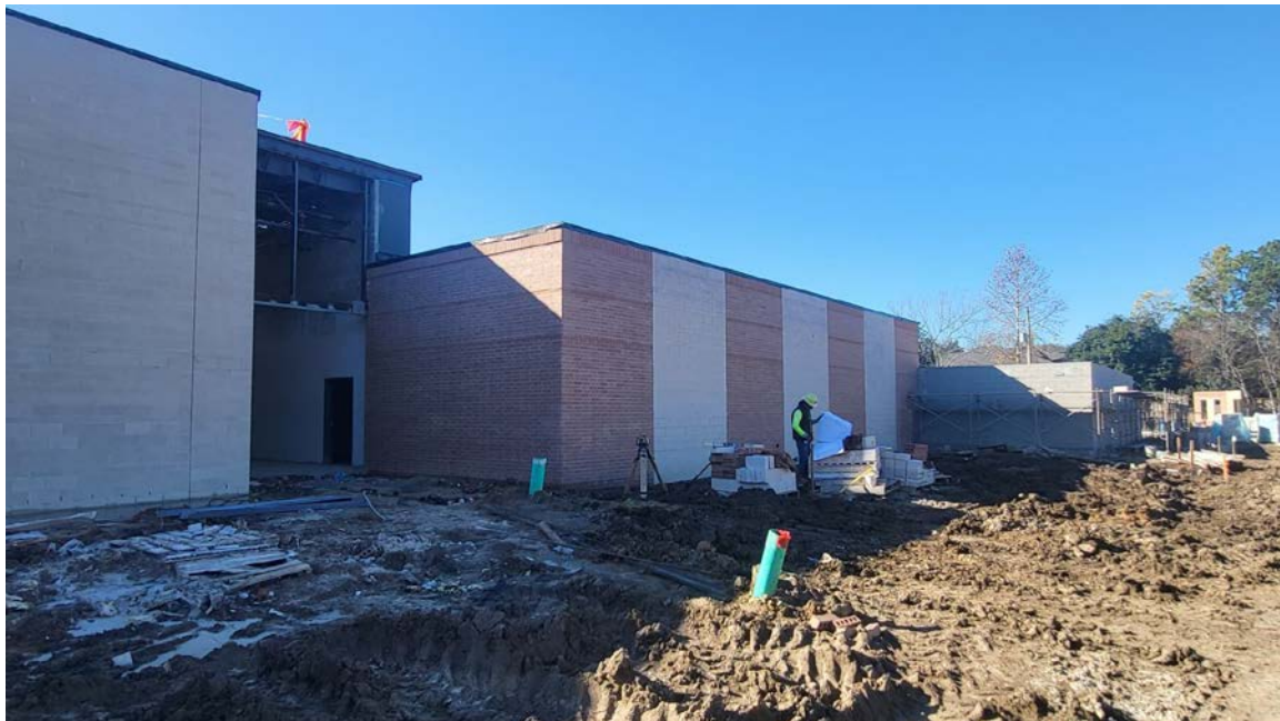
Area F Masonry at North Elevation
