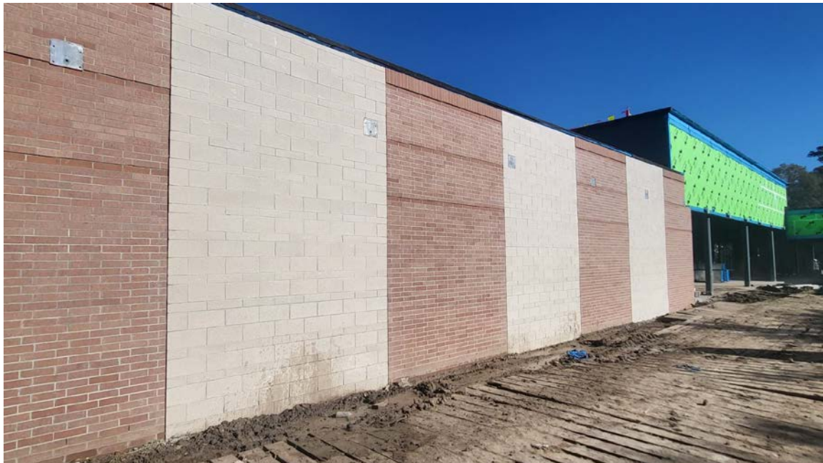
Masonry at Area F South Elevation in Courtyard
