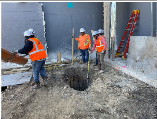
Item #04: Concrete placement for pier at the cafeteria addition.
