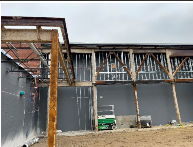
Item #03: Demolition nearly complete at cafeteria addition.
