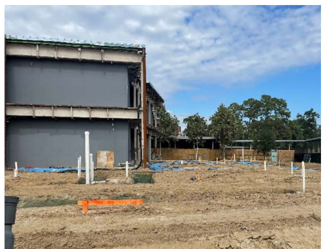
Item #06: Plumbing installation at the classroom addition.
