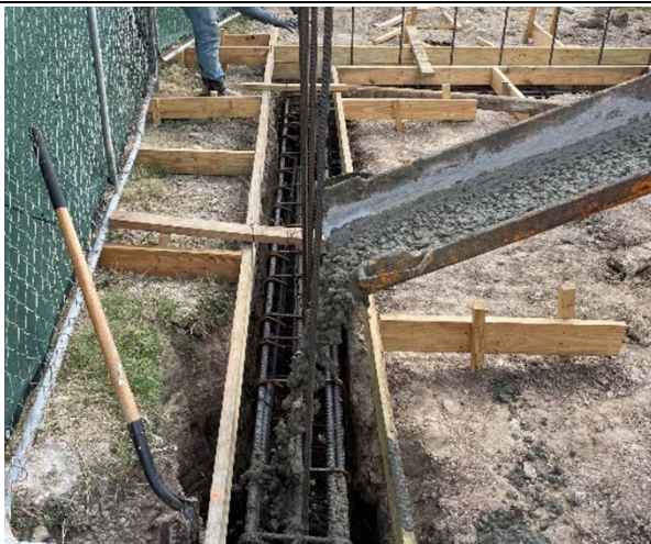
Item #01: Concrete placement of curb at the mechanical yard.
