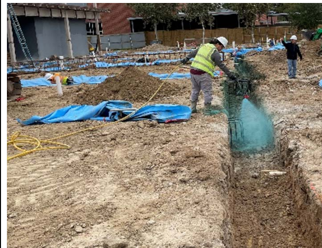
Item #05: Application of termite pest control at the grade beam excavation.
