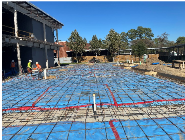
Item #01: SOG formwork, vapor barrier, and reinforcement steel installation.
