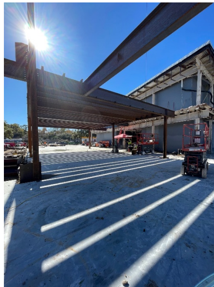
Item #04: View of structural steel erection in the classroom addition area
