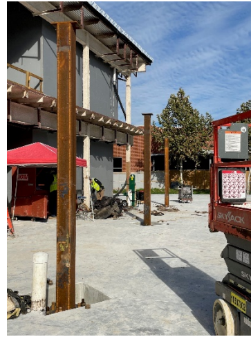
Item #02: Commencement of steel column erection at classroom additional,
