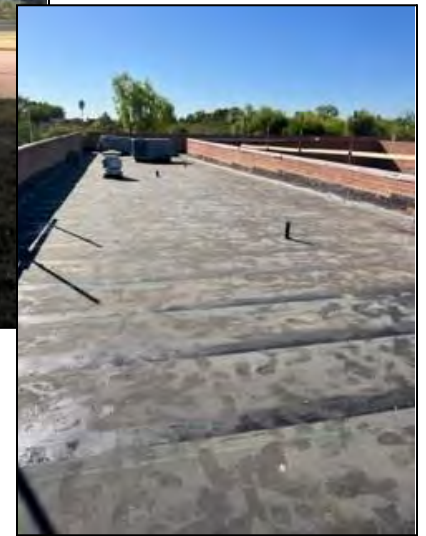
Pueblo Middle School Roof
