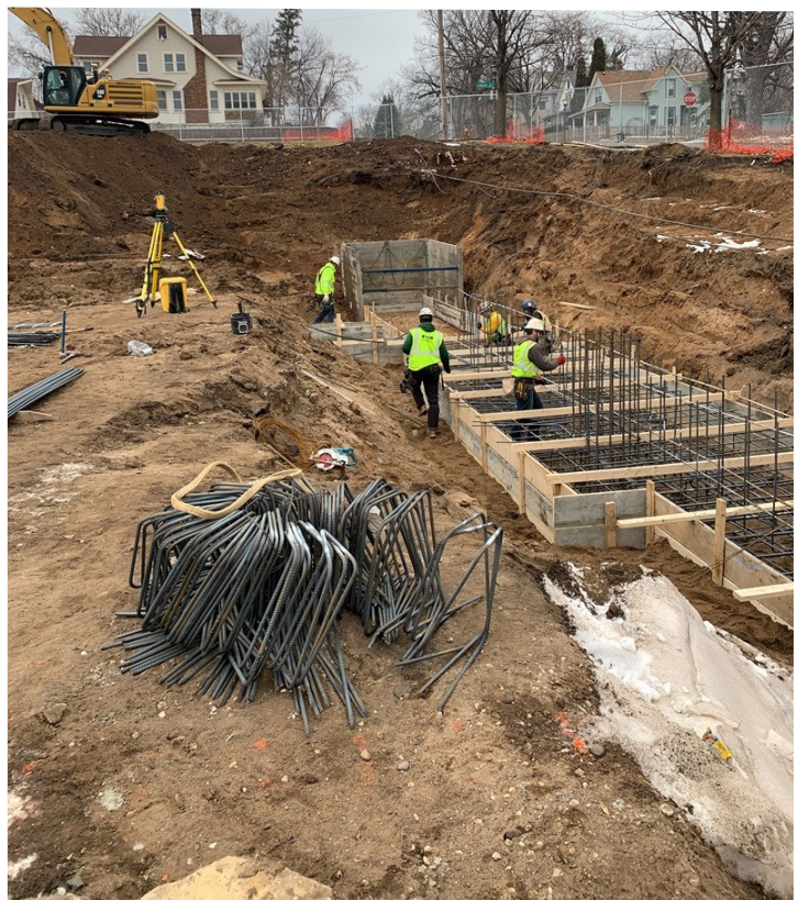
Front top, left to right: Carefully avoiding buried utility lines; digging for footings; forms for east-side concrete walls; setting rebar (January 2024)
