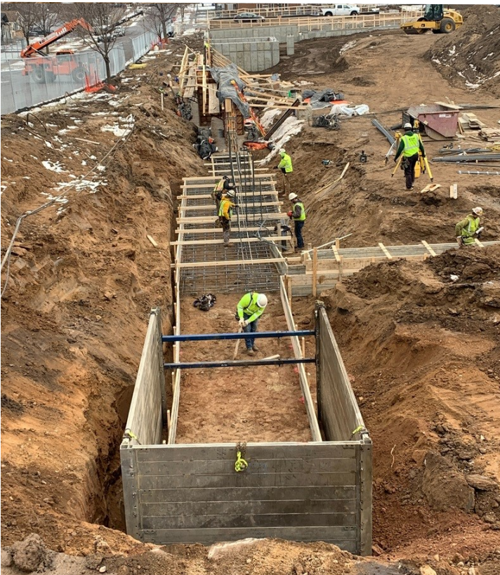
Front top, left to right: Carefully avoiding buried utility lines; digging for footings; forms for east-side concrete walls; setting rebar (January 2024)
