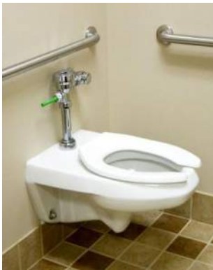
Dual flush toilets and infrared faucets installed at Elgin Academy in Elgin.
