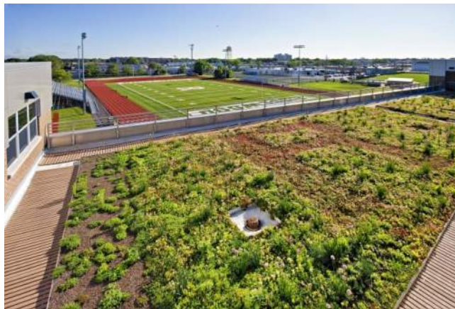
Green roof at Ridgewood High School in Norridge, IL.
