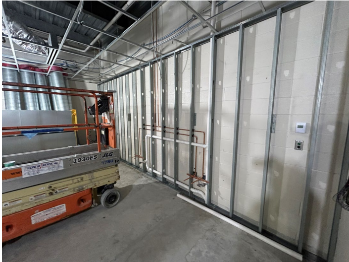
Metal Stud Framing in 3D Art Room
