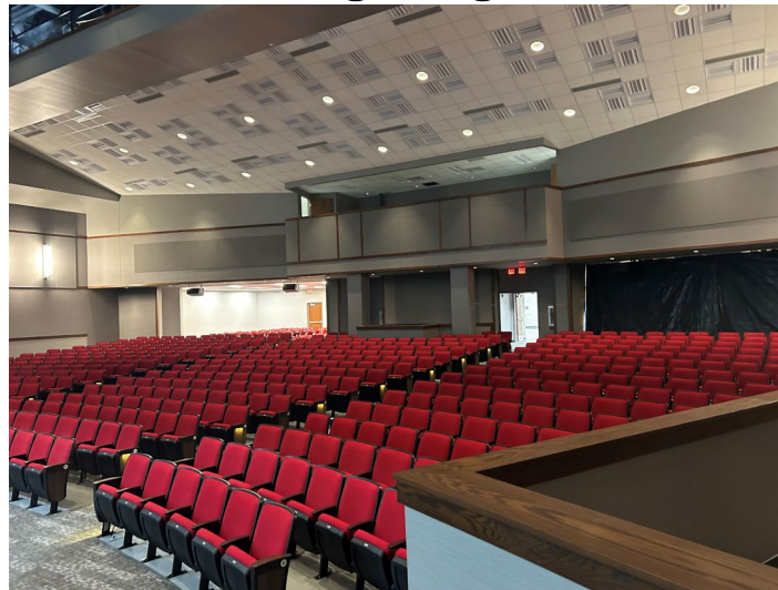
New Auditorium Lighting
