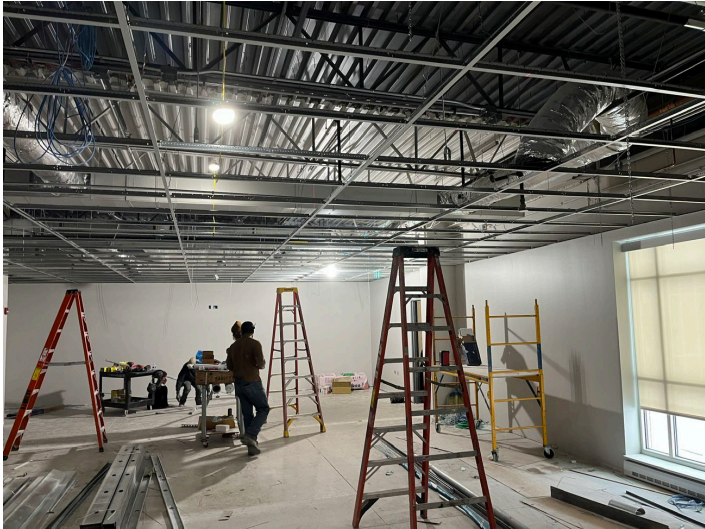
Ceiling Grid in Unit H
