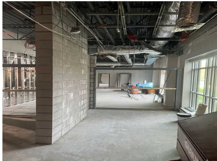
Corridor Doors in Learning Center
