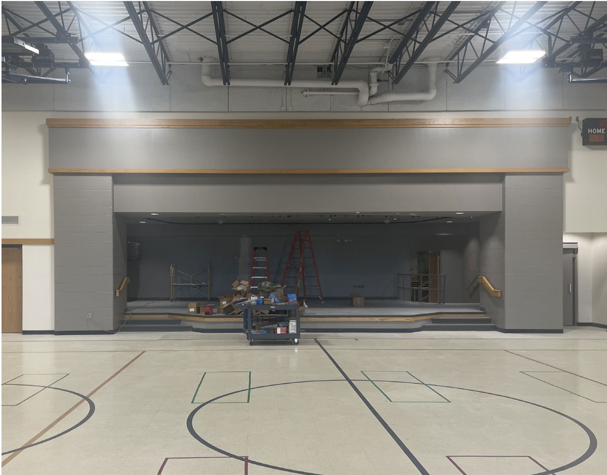
New Stage in Gymnasium
