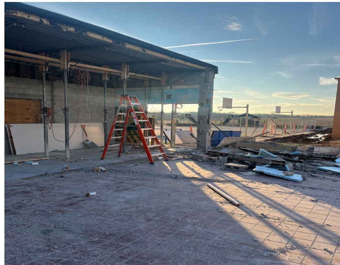
Old Kitchen Demolition
