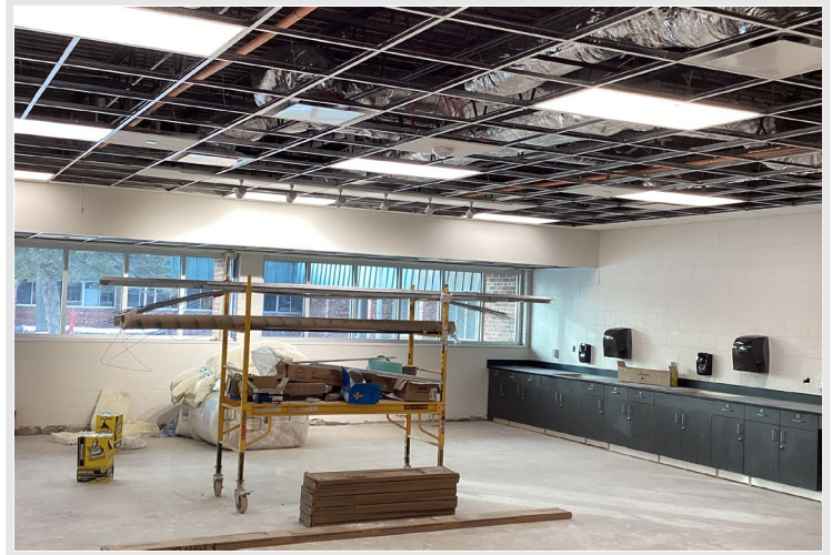
Cabinetry and ceiling grid installation continues in the new art spaces
