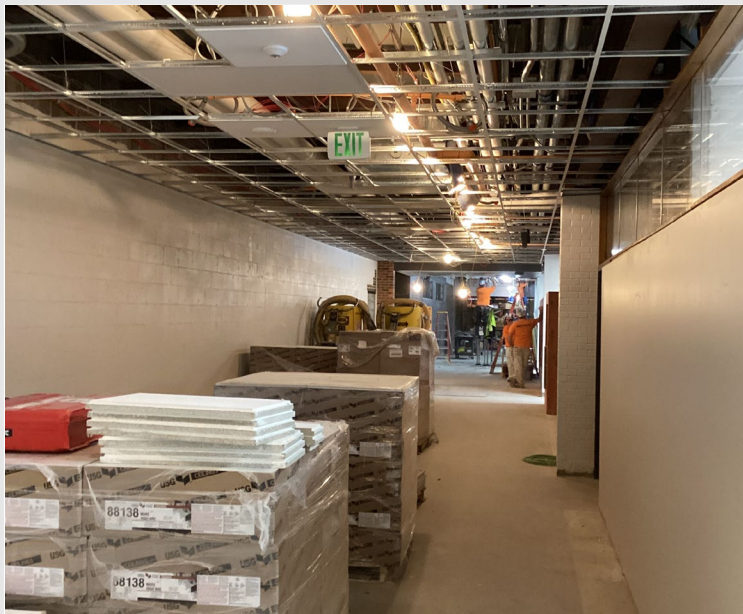
Ceiling grid installation is in progress in the art wing corridor
