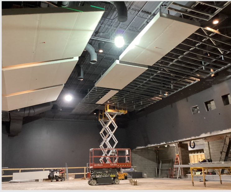
Ceiling clouds are being installed in the PAC
