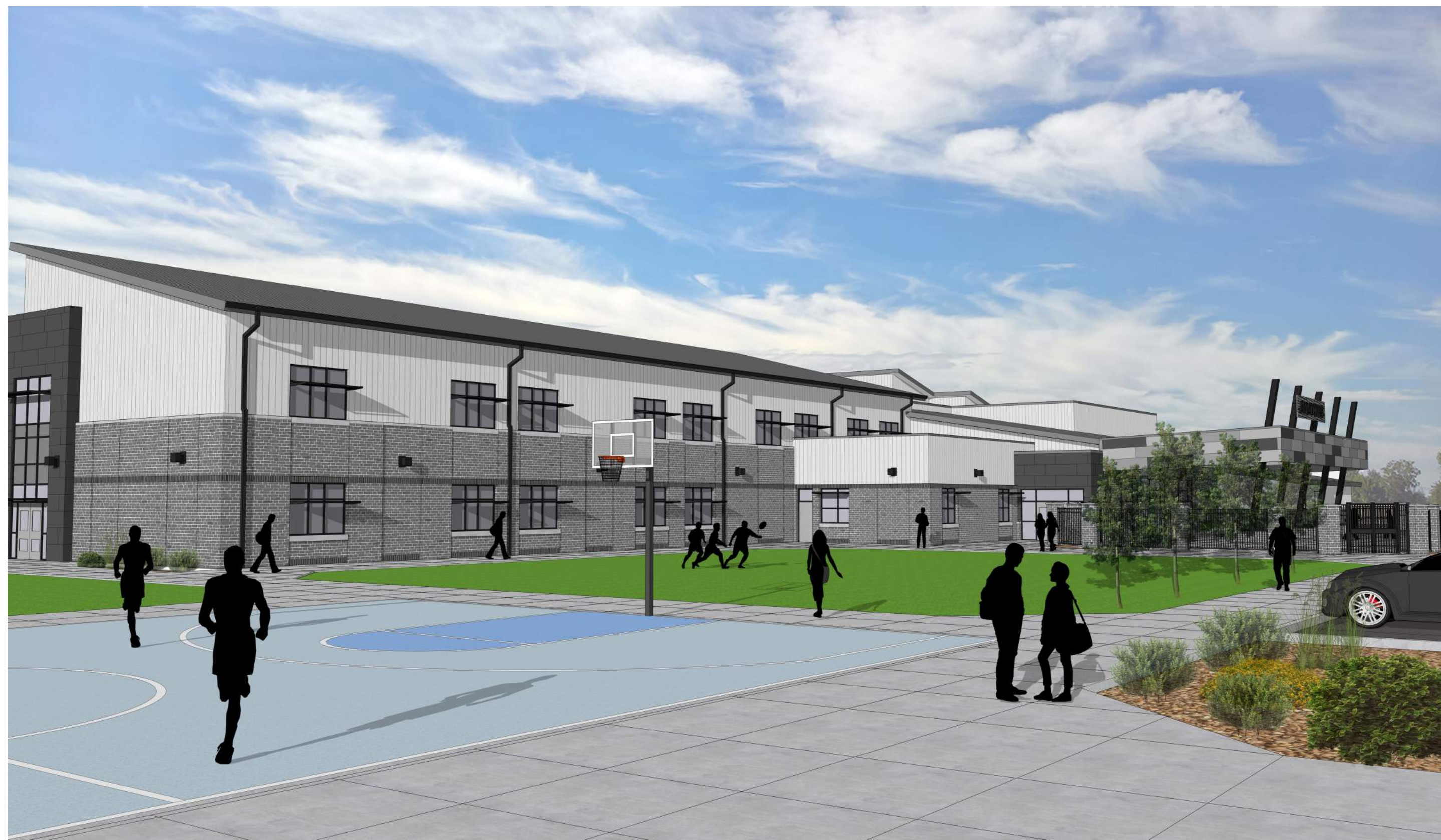
SOUTH WEST VIEW
