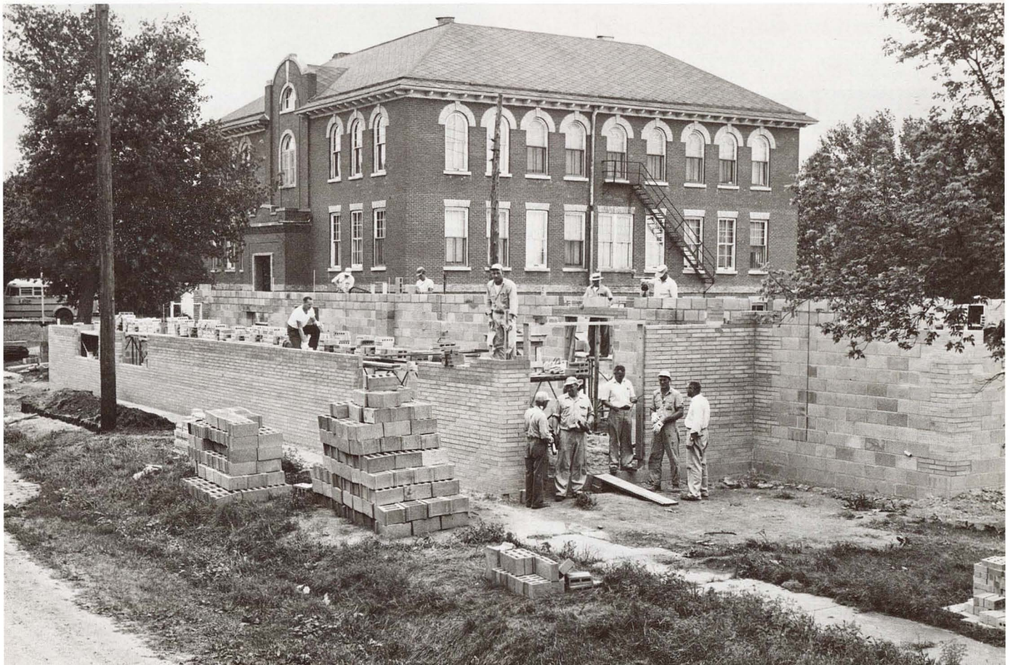
Gary School, 1957, Addition in progress.
