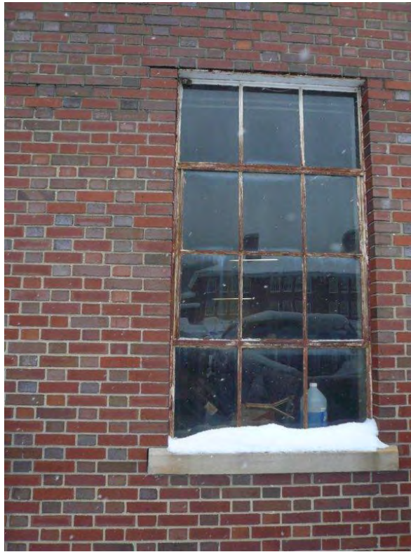
Maint. Facility – Replace steel windows
