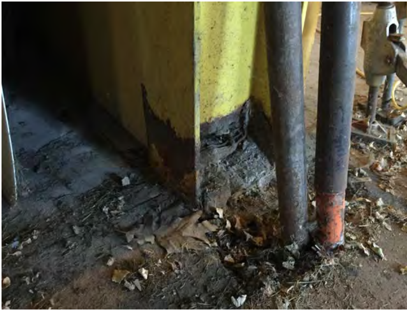
Maint. Facility – Repair column bases
