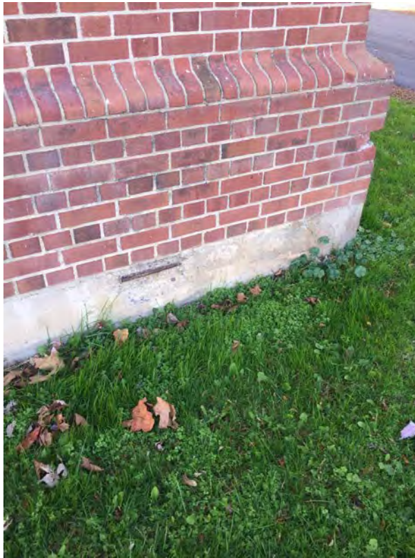
KCH – Masonry restoration, spalled foundation
