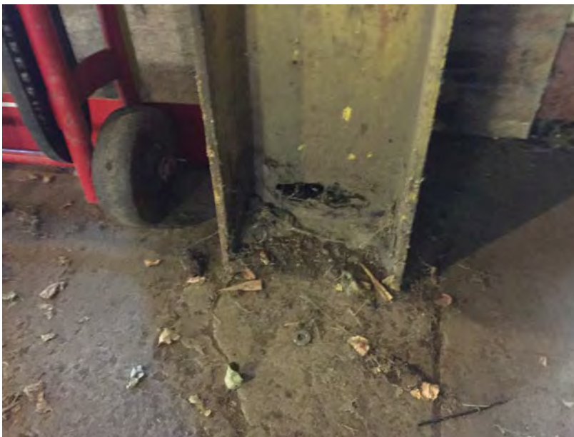
Maint. Facility – Repair column bases
