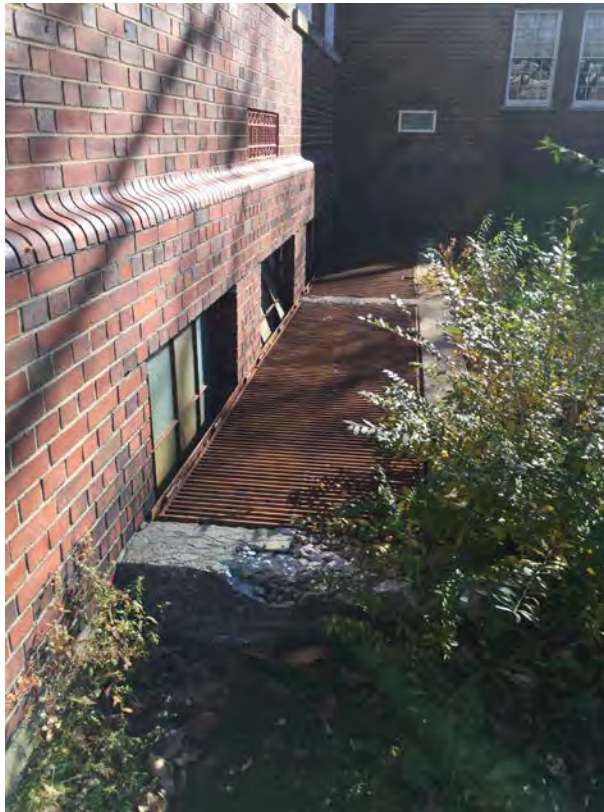
DMS – Courtyard areaway deterioration
