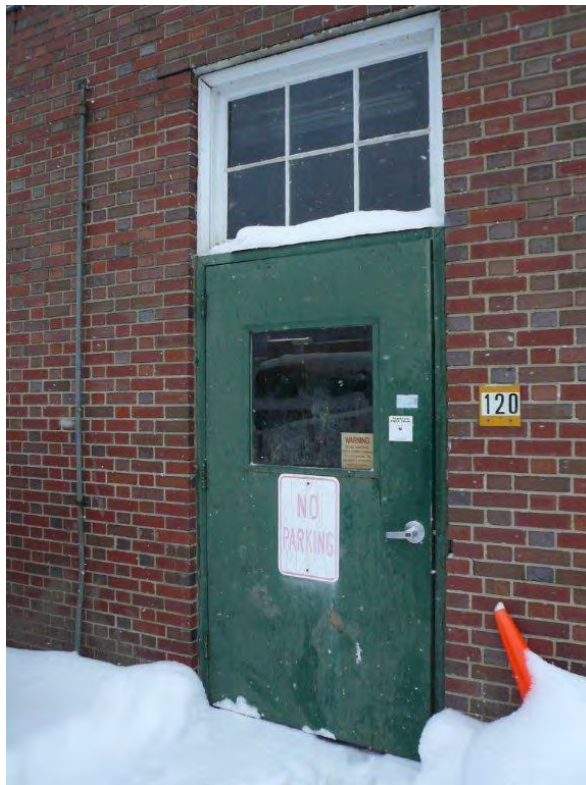
Maint. Facility – Replace exterior man doors
