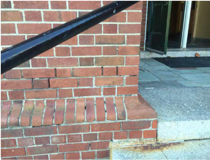
KCH – Mortar deterioration
