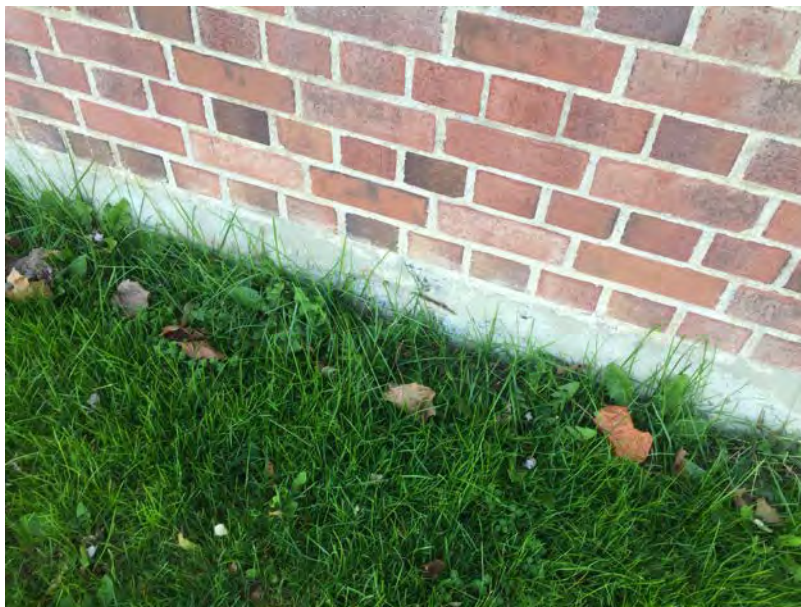
KCH – Masonry restoration, spalled foundation
