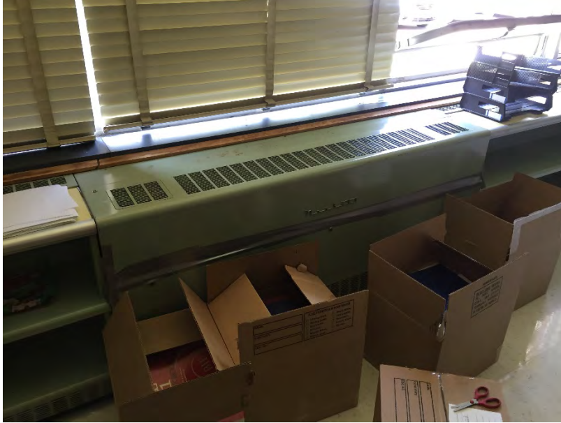
KES - Replace terminal units / heat piping
