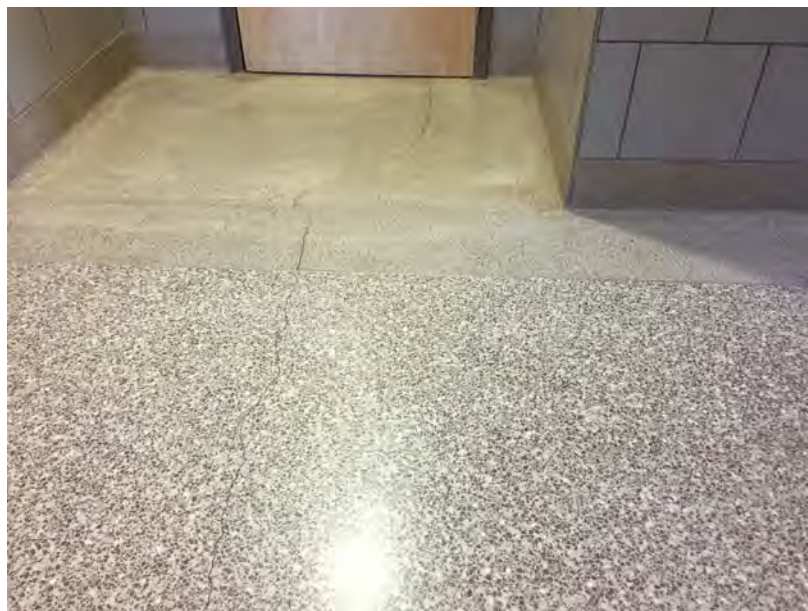
DMS – Resolve floor cracks in newer additions
