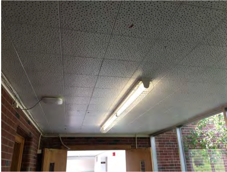
KES – Replace concealed spline ceilings and lighting
